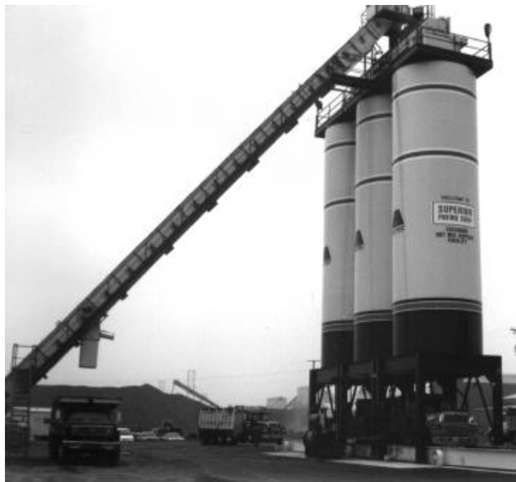
Figure 11.8 Slat conveyor feeding silos at a hot mix plant.
