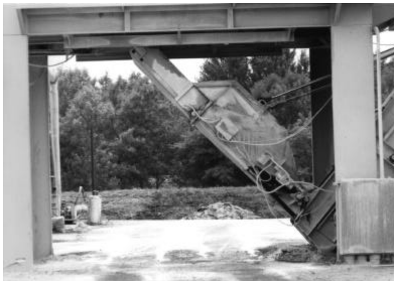
Figure 11.12 Knuckle chute in position to receive mix.
