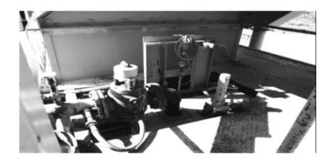
Figure 4.22 Asphalt fill valve on batch tower.
