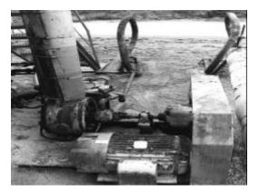
Figure 4.17 Asphalt tank off-loading pump.
