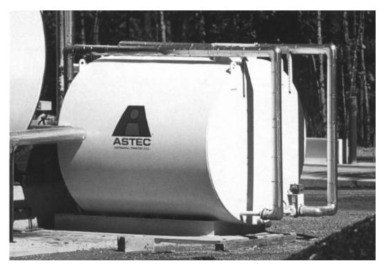
Figure 4.30 Liquid asphalt binder additive tank system.
