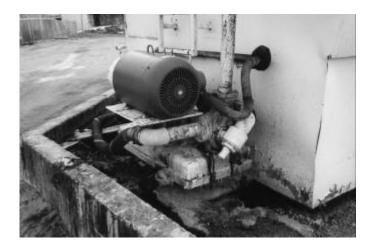
Figure 4.21 Asphalt pump with hot oil lines attached.
