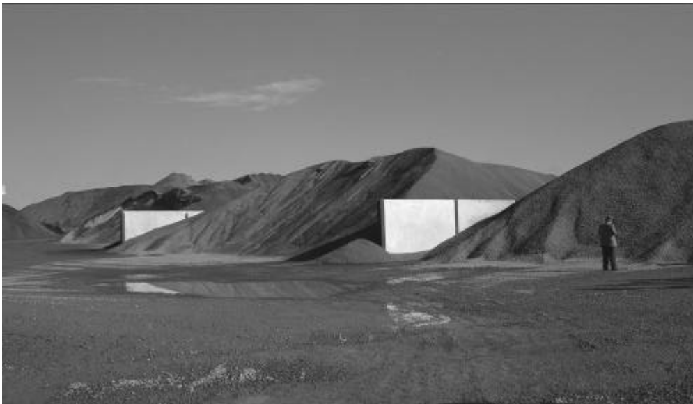
Figure 3.9 Bunker storage used with truck delivery.
