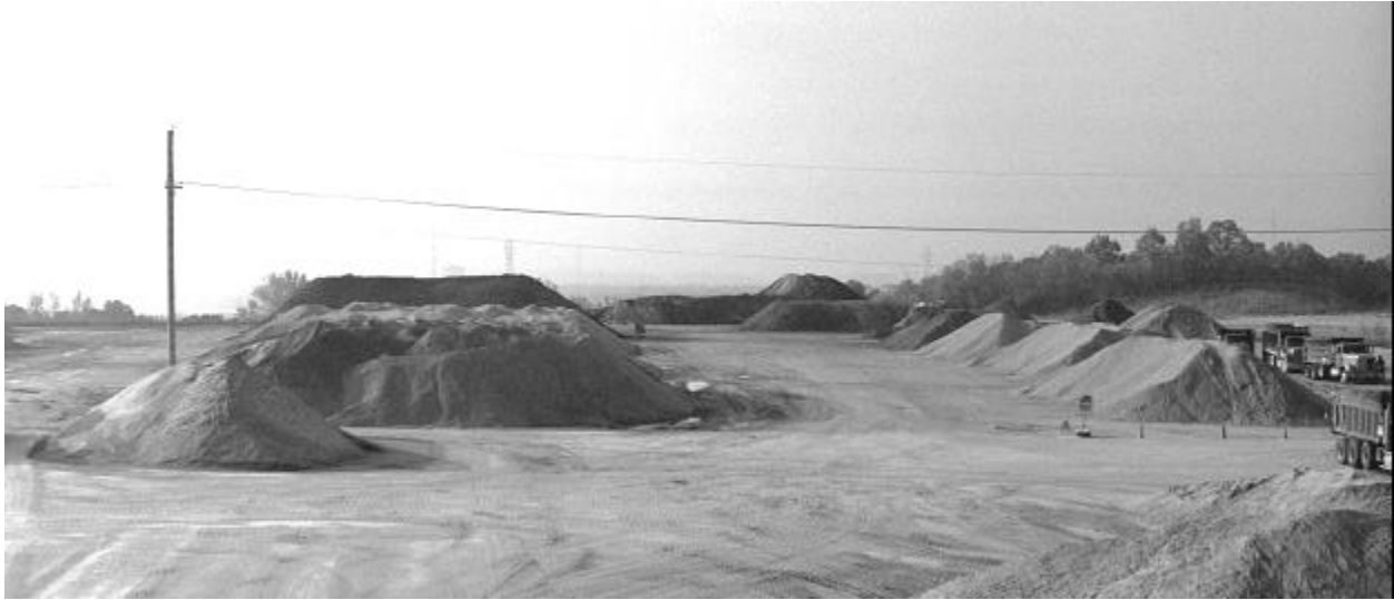
Figure 3.2 Horizontally stockpiling with properly separated aggregate piles.
