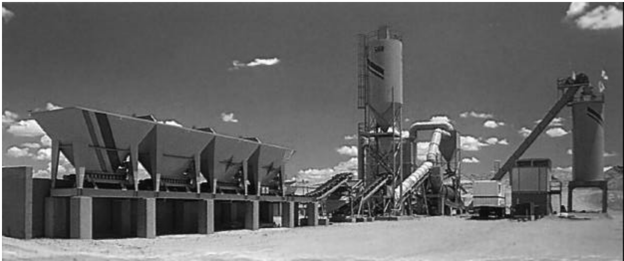
Figure 3.24 Drum-mixer with feeder belts on cold feed bins.
