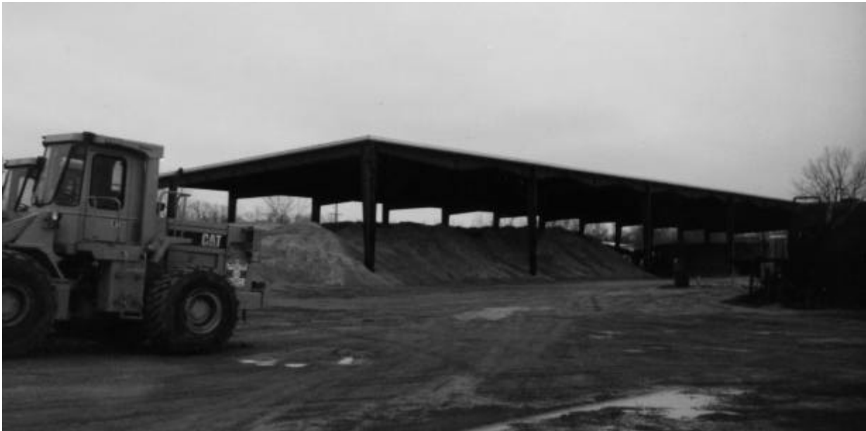
Figure 3.4 Covered aggregate stockpiles.
