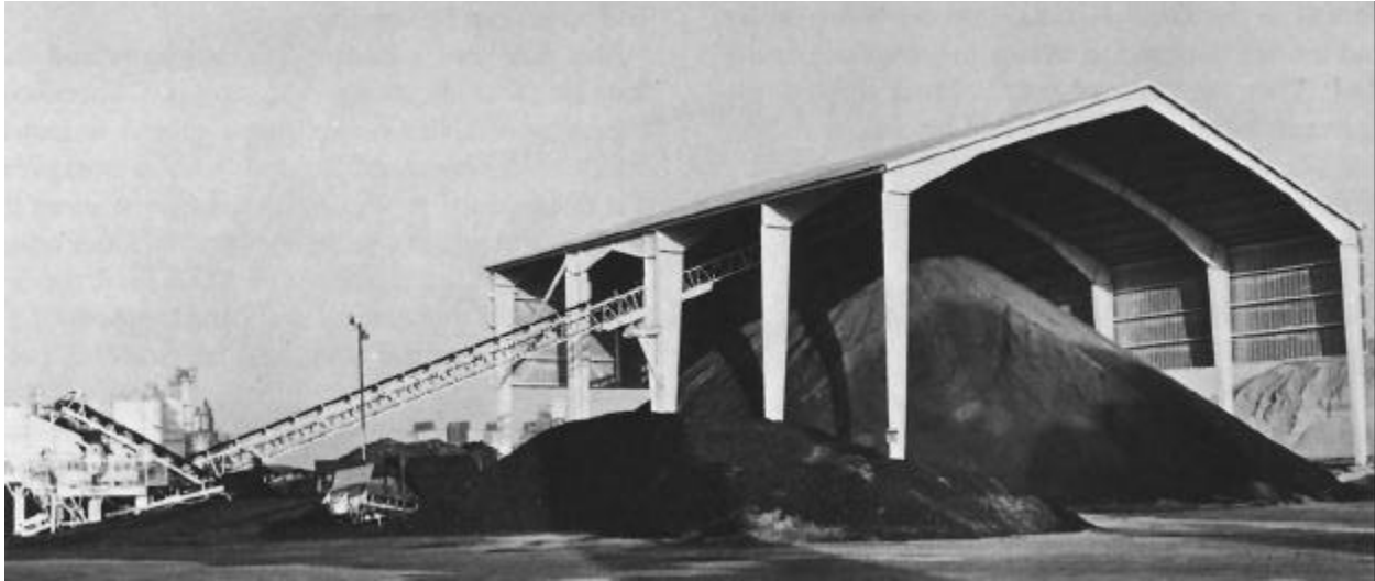
Figure 3.19 Covered RAP stockpile.
