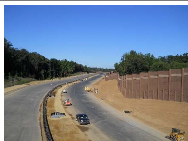
Looking west from Redland Road Bridge with completed noise wall
