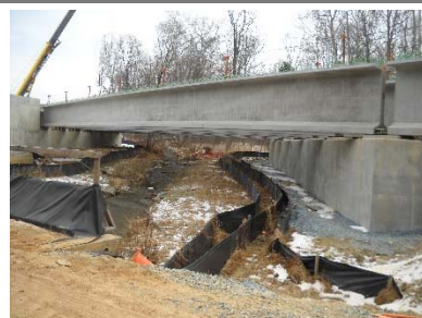
New bridge over stream with redundant E&SC
