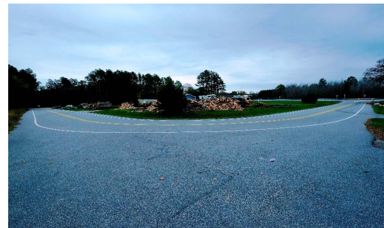
The Service Road installed off MD 404
