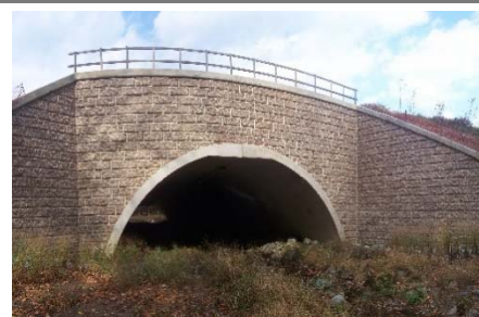
Open Bottom culvert to maintain natural stream bed
