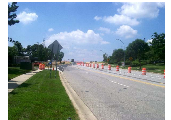
Widening of Sweitzer Lane
