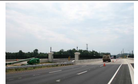
Southbound view of Georgia Ave. Bridge
