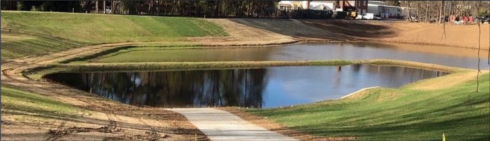
Carroll County Langdon Stormwater Management Facility
