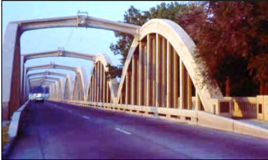
Figure 7. A crash tested traffic railing that blends well with many historic bridges is the Kansas coral railing, used here on the John Mack Bridge at Wichita, KS. Adding it to the historic bridge was no adverse effect.
