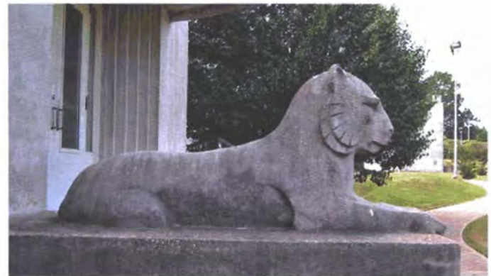
Figure 7. Detailed bas reliefs as well as sculptures, such as this lion at the Bailey Magnet School, could be used as ornamentation on concrete buildings. Sculptural concrete elements were typically cast in molds.
