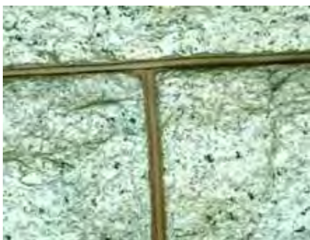
This late 19th century granite has recently been repointed with the joint profile and mortar color carefully matched to the original. Photo: NPS files.
