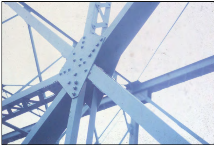
Figure 3 (left). Modern steel bars with end eyes that will fit around the original pins in the same manner and configuration of the members they are replacing.
