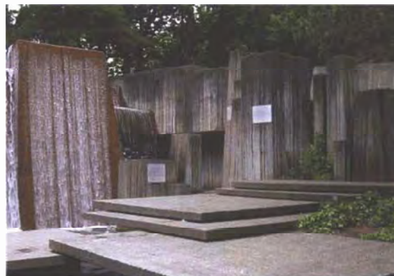
Figure 9. The Ira C. Keller Fountain in Portland, Oregon, was designed by Lawrence Halprin and constructed in 1969. The fountain is constructed primarily of concrete pillars with formboard textures and surrounding elements, patterned with geometric lines, which facilitate the path of water. Photo: Anita Washko, Wiss, Janney, Elstner Associates, Inc.
