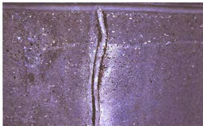
Figure 19. A high-speed grinder is used to widen a crack in preparation for installation of a sealant. This process is called "routing." After the crack is prepared, the sealant is installed to prevent moisture infiltration through the crack. Although sealant repairs can provide a durable, watertight repair for moving cracks, they tend to be very visible.
