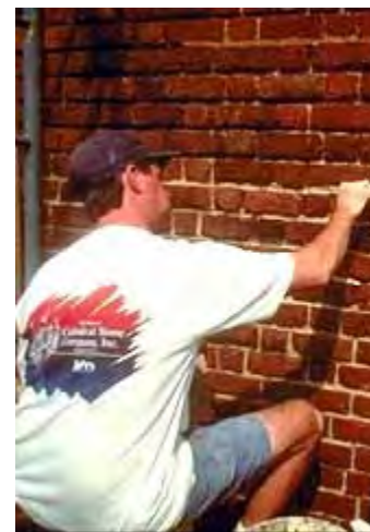
This early 19th century building is being repointed with lime mortar. Photo: Travis McDonald.
