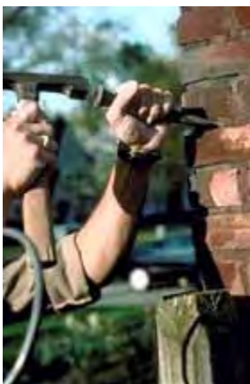
Here, a hammer and chisel are being correctly
