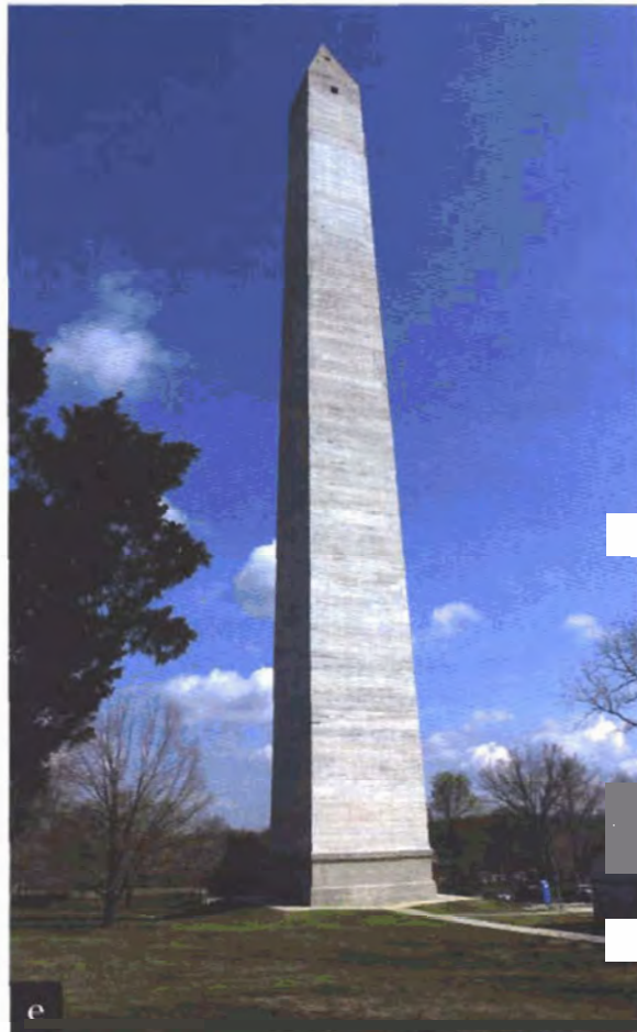
Figure 20. (a) The Jefferson Davis Memorial in Fairview, Kentucky, constructed from 1917–1924, is 351 feet tall and constructed of unreinforced concrete. The walls of the memorial are 8 feet thick at the base and 2 feet thick at the top of the wall. Access to the monument for investigation was provided by rappelling techniques, while ground supported and suspended scaffolding was used to access the exterior during repairs. (b) The concrete was severely deteriorated at isolated locations, with spalling and damage from cyclic freezing and thawing of entrapped water. In addition, previous repairs were at the end of their service life and removal of deteriorated concrete and failed previous repairs was required. Light duty chipping hammers were used to avoid damage to adjacent material when removing deteriorated concrete to the level of sound concrete. (c) Field samples were performed to match the color, finish, and texture of the original concrete. A challenge in matching of historic concrete is achieving variability of appearance. (d) The completed surface after repairs exhibits intentional variability of the concrete surface to match the appearance of the original concrete. Some formwork imperfections that would normally be removed by finishing were intentionally left in place, to replicate the highly variable finish of the original concrete. (e) The Jefferson Davis Memorial after completion of repairs in 2004. Photo e: Joseph Lenzi, Senler, Campbell & Associates, Inc.
