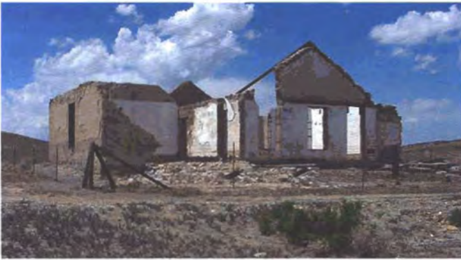
Figure 2. Chatterton House was the home of the post trader at Fort Fred Steel in Wyoming, one of several forts established in the 1860s to protect the Union Pacific Railroad. The walls of the post trader's house were built using stone aggregate and lime, without cement. The use of this material presents special preservation challenges.
