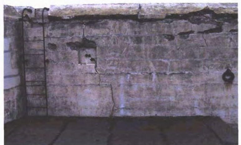
Figure 13. Fort Casey on Admiralty Head, Fort Casey, Washington, was constructed in 1898. The lift lines from placement of concrete are clearly visible on the exterior walls and characterize the finished appearance.
