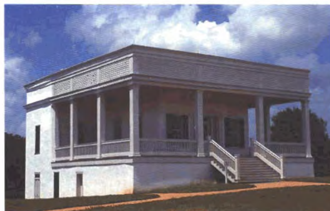
Figure 1. The Sebastopol House in Seguin, Texas, is an 1856 Greek Revival-style house constructed of lime concrete. Lime concrete or "limecrete" was a popular construction material, as it could be made inexpensively from local materials. By 1900, the town had approximately ninety limecrete structures, twenty of which remain. Photo: Texas Parks and Wildlife Department.
