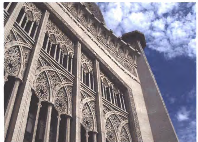
Figure 4. The highly ornamental concrete panels on the exterior facade of the Baha'i House of Worship in Wilmette, Illinois, illustrate the work of fabricator John J. Earley, known as "the man who made concrete beautiful."
