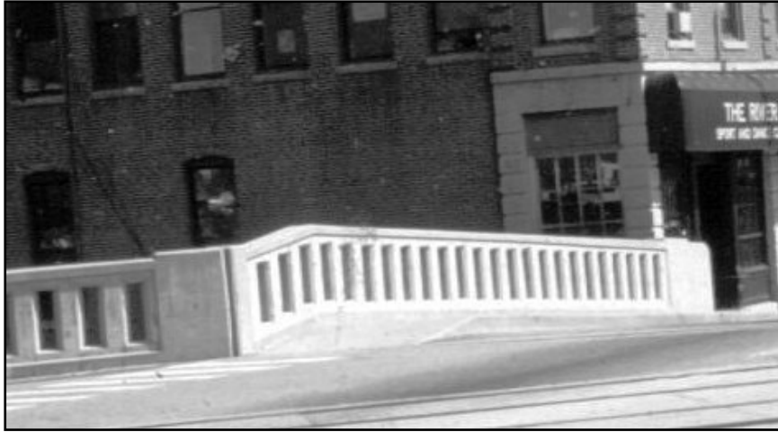
Figure 9. This is an appropriate, urban use of the crash-tested Texas Railing. It has proven to be a good replacement design for open balustrade railings used by many departments of transportation through the 1950s. This railing would not be appropriate for a rural setting because historically it was rarely used for non-urban bridges.
