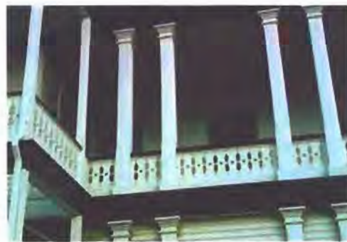
Decorative wood exterior or interior features should not be cleaned abrasively. Photo: NPS files.
