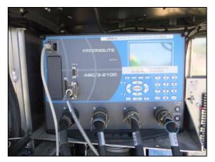
Figure SG. 36 - Signal Controller
