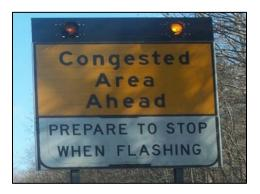
Figure SG. 12 - HIB Mounted within Sign Panel
