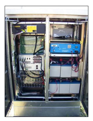
Figure SG. 39 - Typical Signal Cabinet with UPS (Size 'S')
