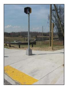
Figure SG. 30 - Acceptable Placement of APS
