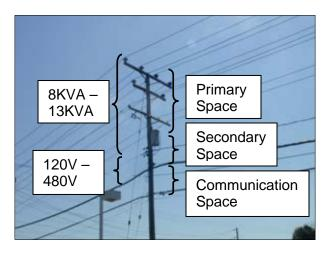
Figure SG. 2 - Typical Utility Pole "Spaces"
