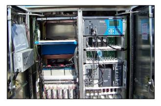
Figure SG. 38 - Typical Signal Cabinet (Size 'S')
