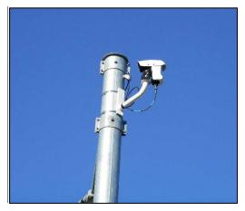
Figure SG. 25 - Typical Video Detection Location (Extension Arm Mount)
