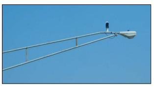
Figure SG. 24 - Typical Video Detection Location (Lighting Arm Mount)
