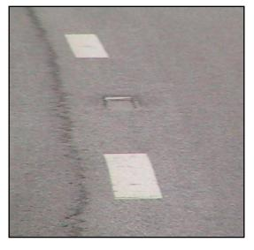
Figure SN.46 - Recessed Pavement Marker (RPM)
