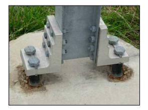
Figure SN. 26 - Breakaway Steel Support
