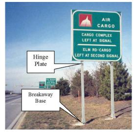
Figure SN.31 - Breakaway Steel Support
