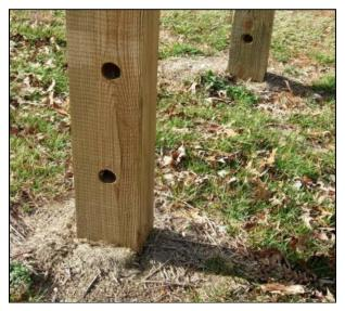
Figure SN.23 - Breakaway Wood Support
