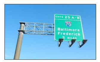
Figure SN.16 - Typical Box Truss Cantilever
