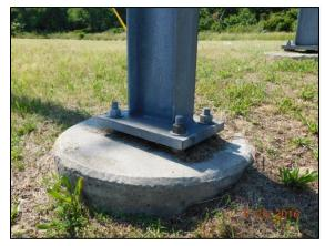
Figure SN. 25 - Non-Breakaway Steel Support
