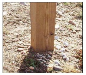
Figure SN.24 - Non-Breakaway Wood Support
