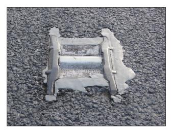
Figure SN.45 – Snowplowable Raised Pavement Marker
