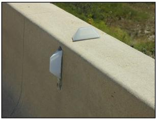
Figure SN.41 - Top and Side Mounted White Barrier Wall Markers
