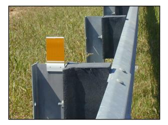
Figure SN.40 - Top Mounted Yellow W-Beam Marker
