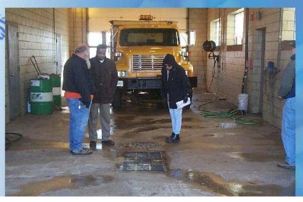
Clean equipment in wash bay so that wash water is treated by the grit separator and oil/water separator to minimize the discharge of sediment, salt and heavy metals into the environment.
