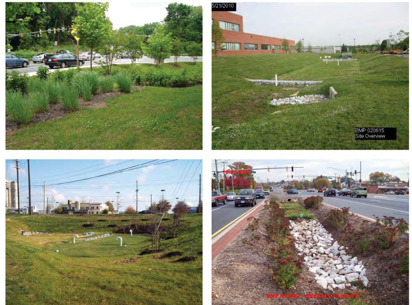
SAMPLE FILTRATION FACILITY PHOTOS
