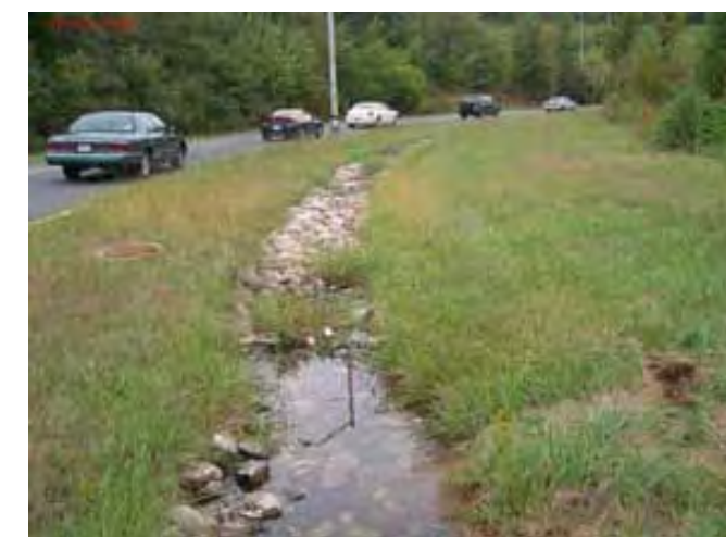
Saturated Infiltration Trench
