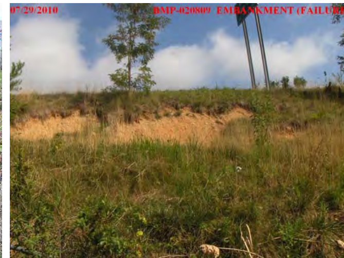
Eroded Embankment
