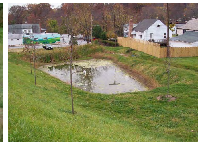
Surface Sand Filter Not Draining
