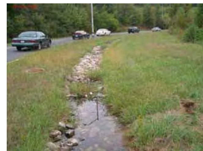
Saturated Infiltration Trench
