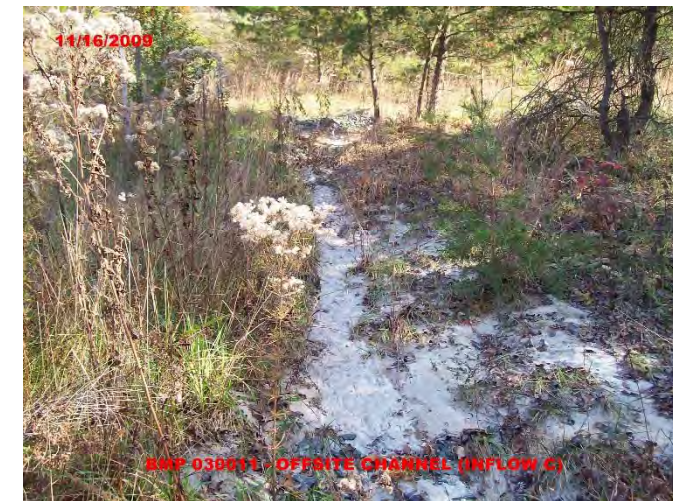
Minor Sediment Accumulation in Inflow Ditch
