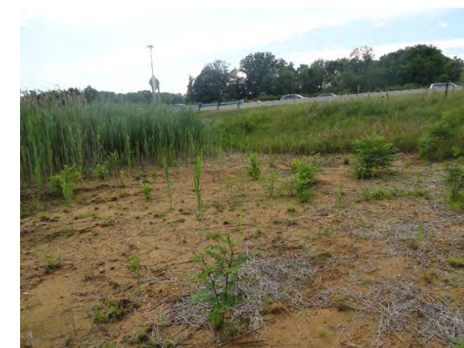
Large Area of Bare Soil on Pond Bottom
