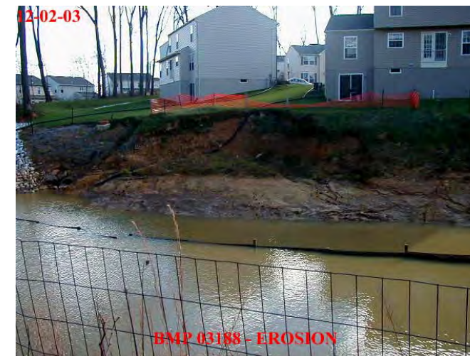
Major Erosion Along Pond Bank
