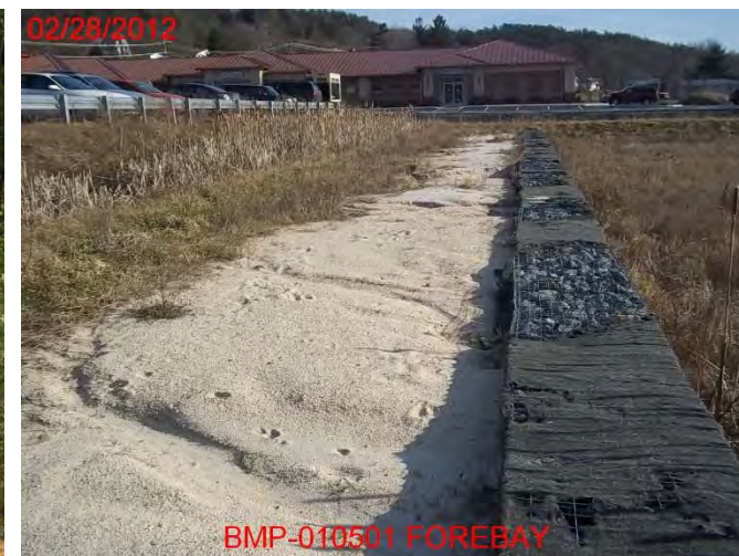
Major Sediment Accumulation in Forebay
