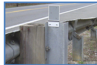
Guardrail with delineator
