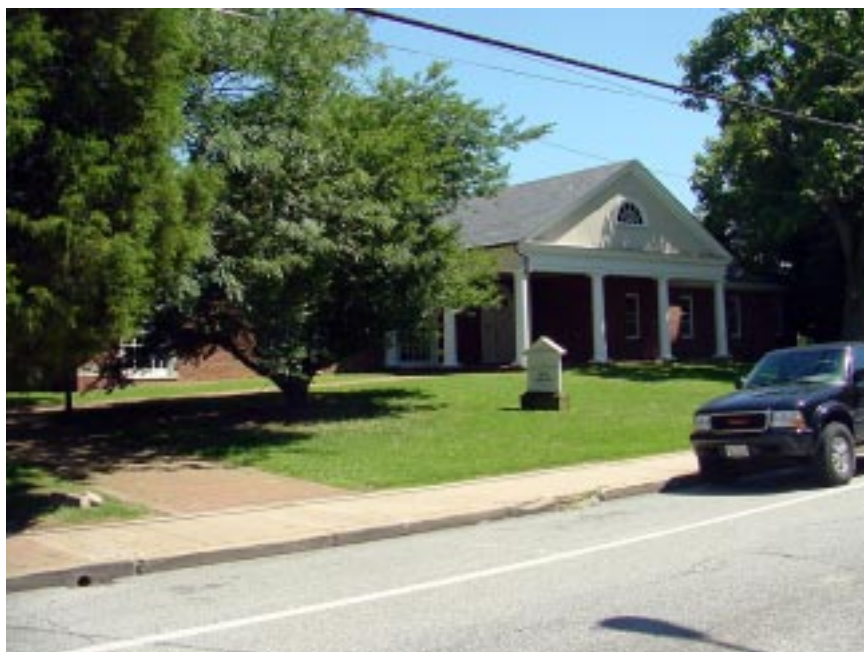
The Queen Anne's County Public Library is a gathering place for county residents and is a great location for installing interpretation about the Byway.
