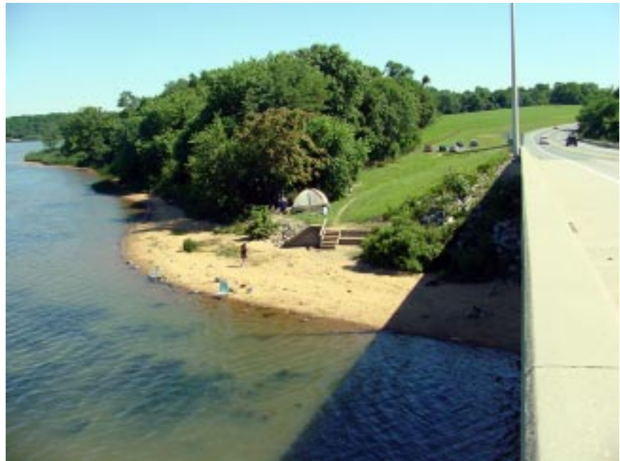
The Bohemia River Landing is a popular spot for water access. Enhancing the site with new walkways, retaining walls, landscaping, and interpretive exhibits is likely to create a popular local destination.
