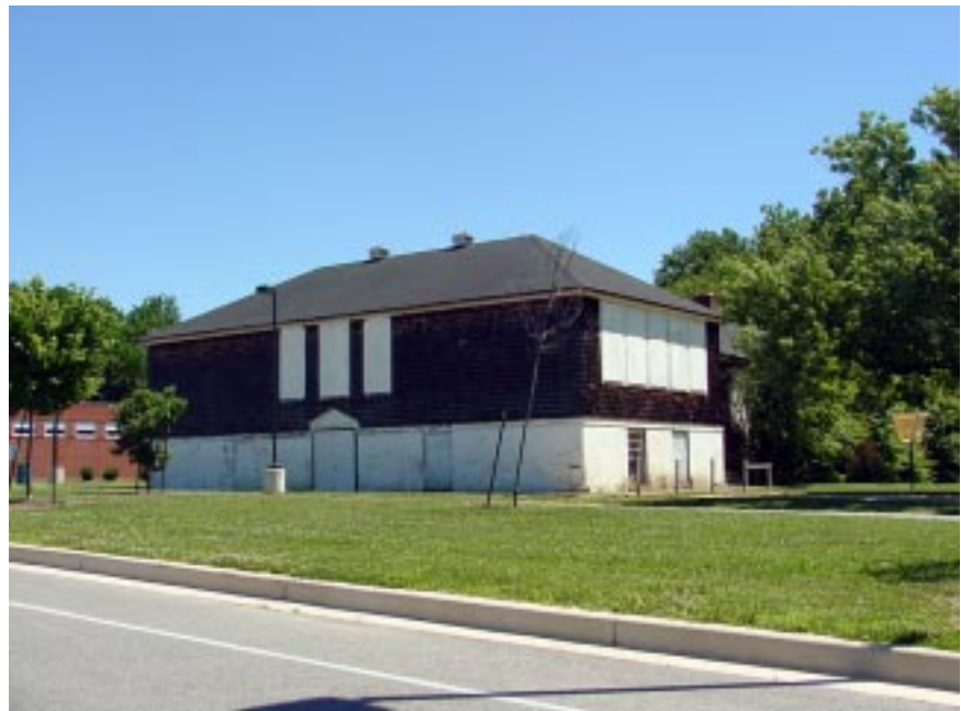
The Kennard School is in great need of rehabilitation. Installation interpretation will help raise awareness and help ensure the longevity of this important structure.
