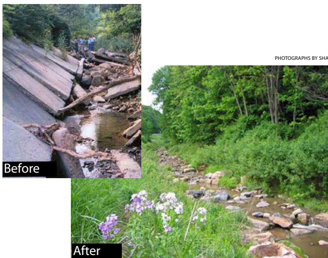
Soil bio-engineering concepts were used by SHA and Maryland Department of Natural Resources to restore Porter Run adjacent to the Historic National Road near Clarysville. Willow whips were interplanted to help stabilize the streambank.
