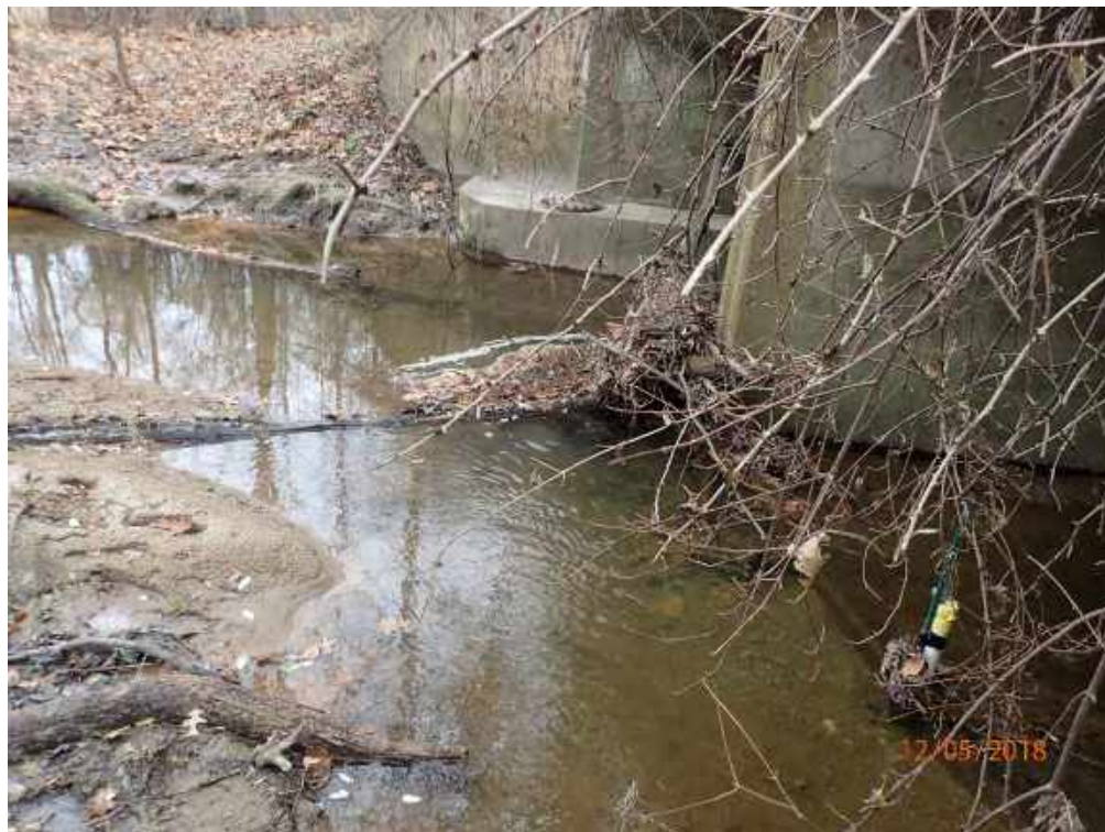
Photograph 66. 12/05/2018: Debris jam at box culvert for Flow Station 1
