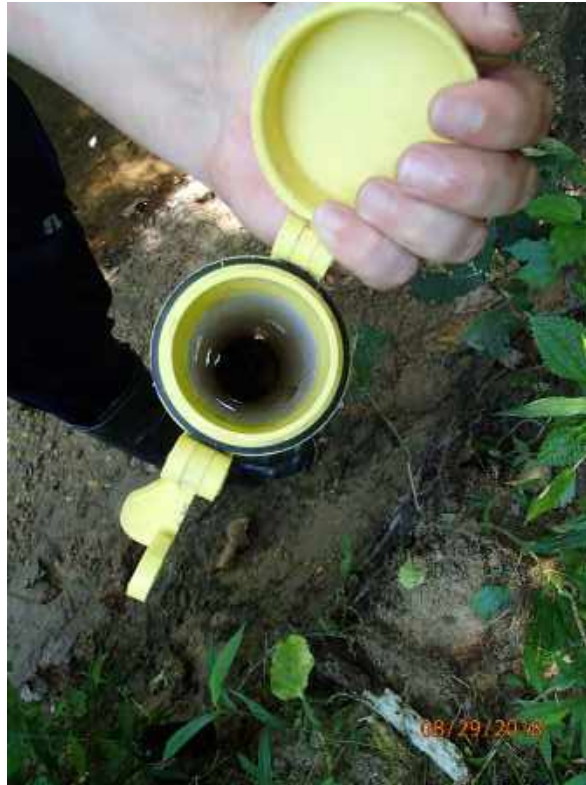
Photograph 18. 8/29/2018: Sediment being cleaned out of Flow Station 1 housing
