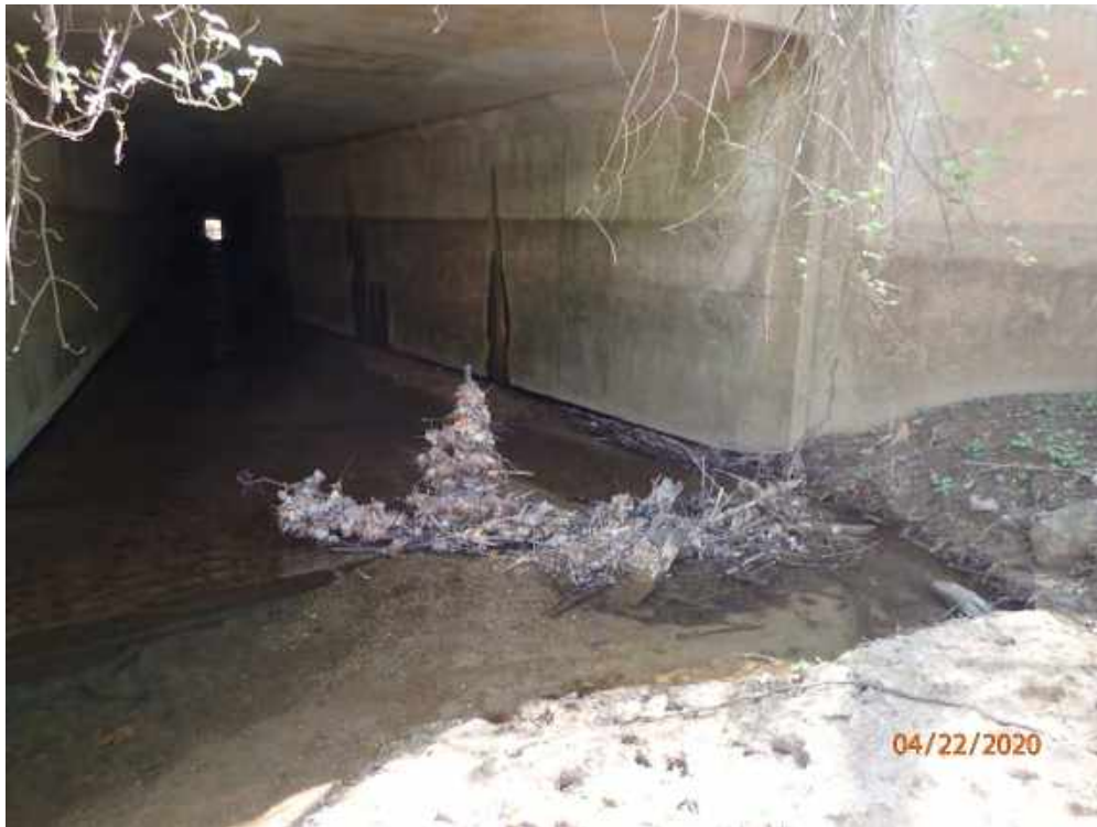
Photograph 148. 4/22/2020: Year 3 Monthly Download and Maintenance, Flow Station 1, dislodged and out of position under weight of debris
