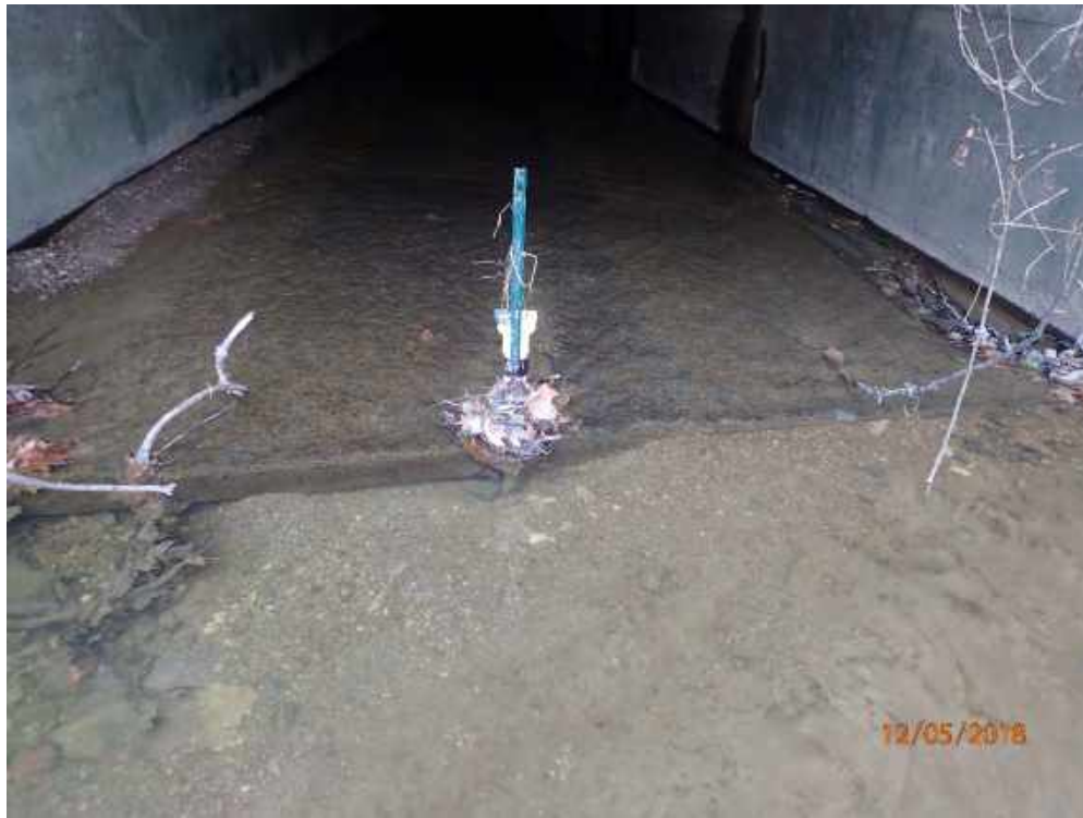
Photograph 66. 12/05/2018: Debris jam at box culvert for Flow Station 1
