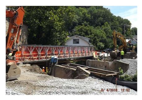
(SHA Photo: MD 222 Bridge over Rock Run. Old bridge is gone and a temporary pedestrian walkway has been installed for access to local businesses. August 2016.)
