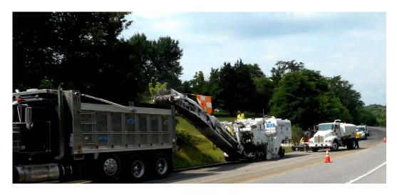
(SHA photo: Crews milling (removing top layer of asphalt) on MD 34 (Shepherdstown Pike in Washington County.)
