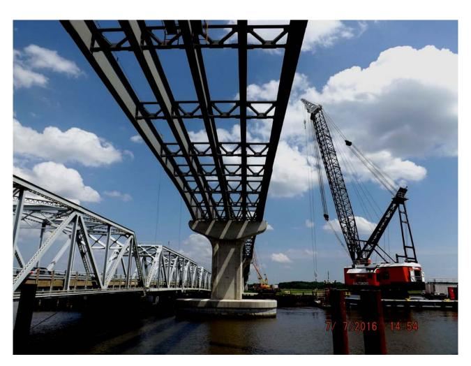
(SHA Photo: Steel beams in place for the new MD 331/Dover Bridge. SHA is pouring concrete bridge deck.)
