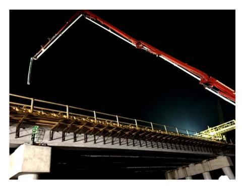
(SHA Photo: Concrete bridge deck pour for the new Dover Bridge project (MD 331 Bridge over Choptank River at the Caroline/Talbot County line. (August 2016)
