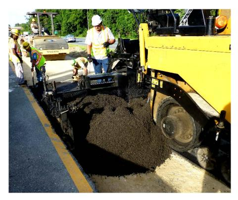
(SHA photo: Widening <u>northbound US 29</u> in Columbia is almost complete. Here, crews are using recycled pavement for the new lane.)
