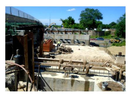
(SHA Photo: Removing old steel beams and demolishing Old Harford Road Bridge over I-695. The new Old Harford Bridge over I-695 opened early-June 2016. This is part of the <u>I-695 between MD 41 (Perring Parkway) and MD 147 (Harford Road)</u>-Widening/Interchange reconstruction)
