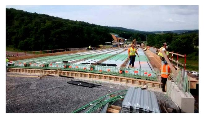
(SHA photo: The MD 546 (Finzel Road) Bridge over I-68. Crews installing new bridge deck (driving surface. Bridge is now opened.)
