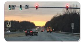
Smart Signals operate with an adaptive signal control system, which uses enhanced detection to monitor traffic conditions and alter the timing of traffic signals. The smart signals will replace existing controls that are over 20 years old and unresponsive to changes in traffic flow, operating instead on programmed timing. This innovative technology quickly considers crashes, construction and congestion, adjusting signal timing accordingly.
