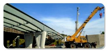
Setting new steel beams for the Old Harford Road Bridge as part of the I-695 between MD 41 and MD 147 interchange reconstruction project
