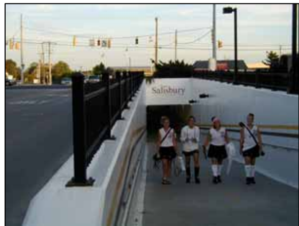
Figure 12.3- Example of an Underpass in Salisbury, MD
