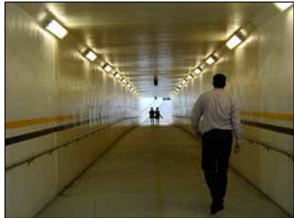
Figure 12.2- Example of Underpass in Salisbury, MD
