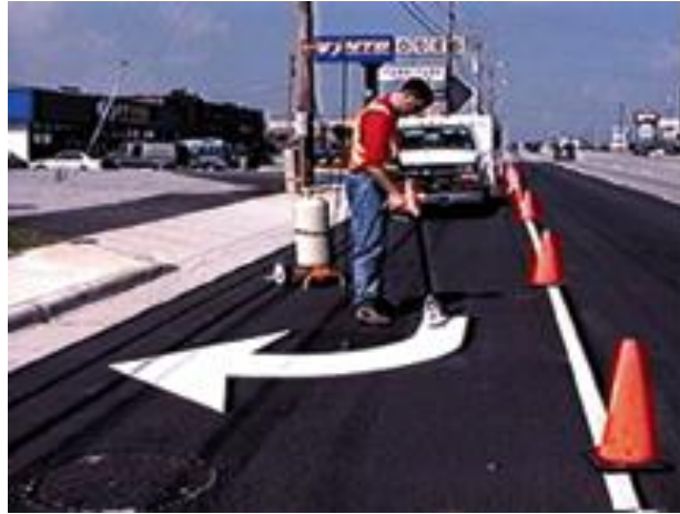
Figure 5.3 Arrow symbol being applied by heat torch.
