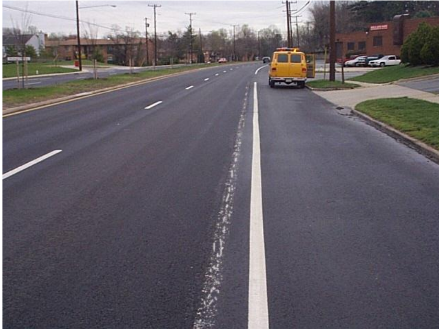
Figure 12.2 Scars from removed marking
