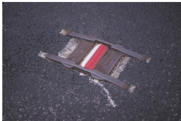
Figure 9.3b Raised, snow plowable marker system shown in-place
