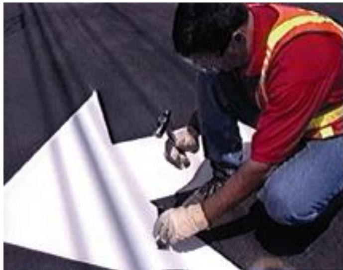
Figure 5.4 Adhesion test being performed
