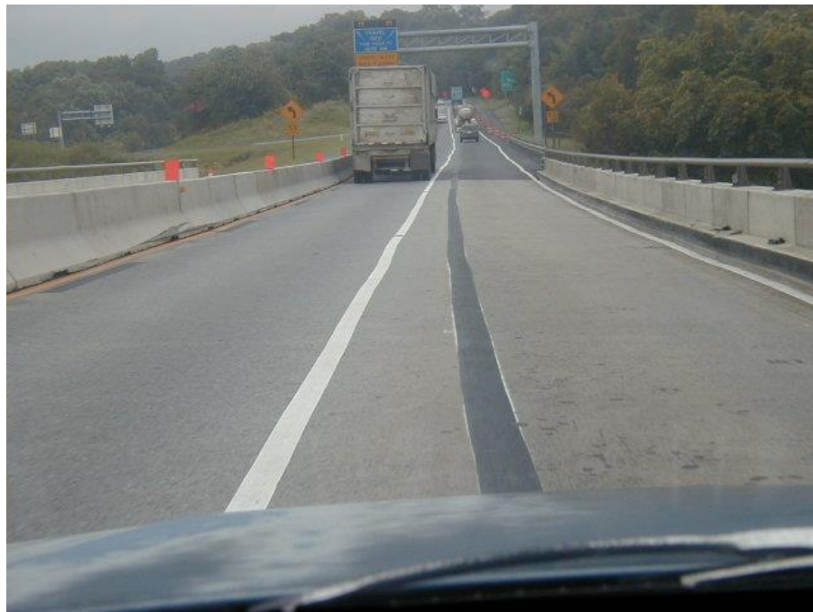
Figure 12.3 Black paint wearing off of previous marking
