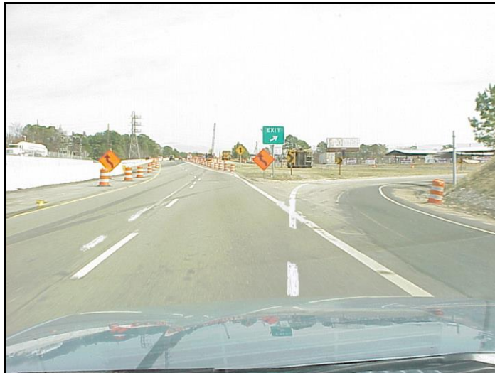
Figure 12.1 Roadway with confusing multiple lines
