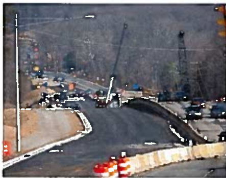
Lane Detour on Route 1
