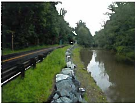
Completed Road and New River Bank
