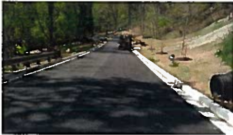
Piscataway Road Paving
