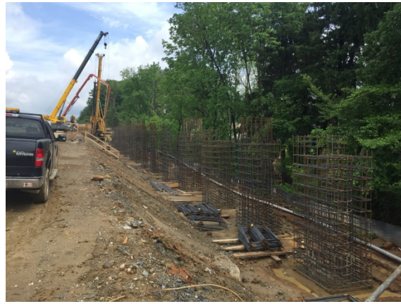
Caissons for IL Noise Barrier looking North
