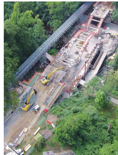
Partial Demolition of the Carroll Avenue Bridge
