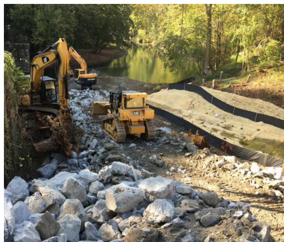
Erosion and Sedimentation Control Measures in Patapsco State Park
