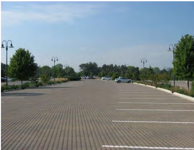
Permeable pavement examples with interlocking pavers and porous bituminous asphalt
