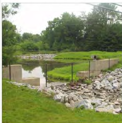
Avoid blocking weir openings with fence as shown above. (See photo to right)
