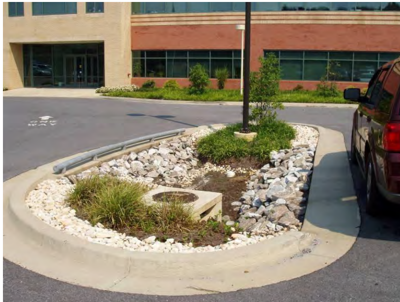
Micro-Bioretention Basin Example
