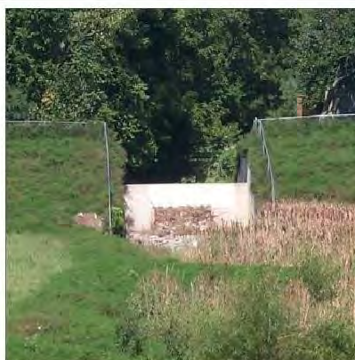
Rather than suspend the fence over this weir structure, the fencing is worked into the design of the structure and embankment.
