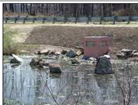
Low Flow Device uses a T-Connection and Runs Parallel to the Side Slopes (Preferred)
