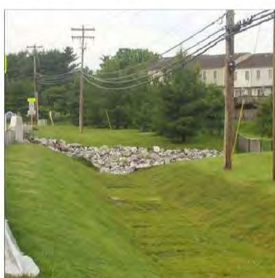
Rather than block the weir opening (left), the fence could have followed along either side of the riprap channel and tied into the endwall. Crossing a ditch farther downstream is preferable to blocking a weir.
