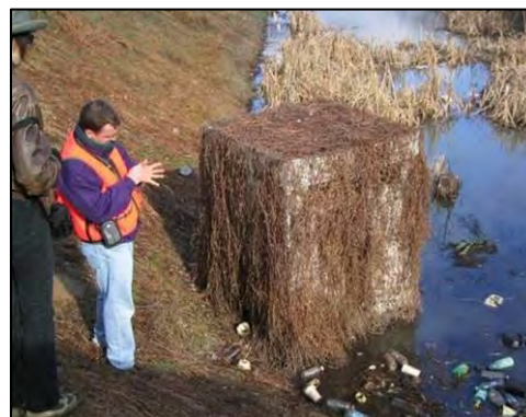
Woody vegetation, including ivy, must be kept clear from a riser structure to ensure proper function.
