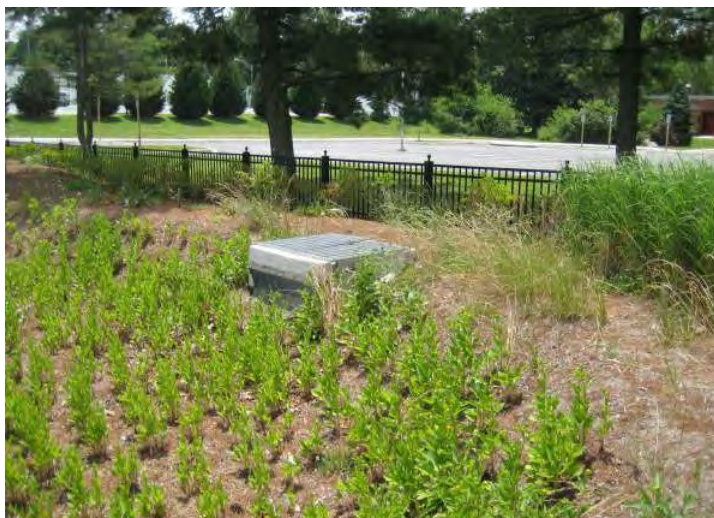
Bioretention Basin Example
