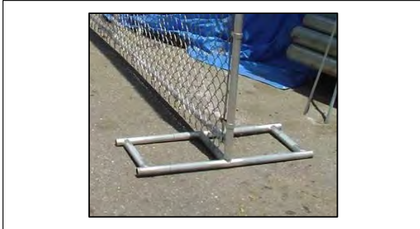
Figure 5-4. Footer at Temporary Fencing
