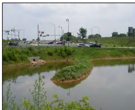
Baffle Constructed from Fill
