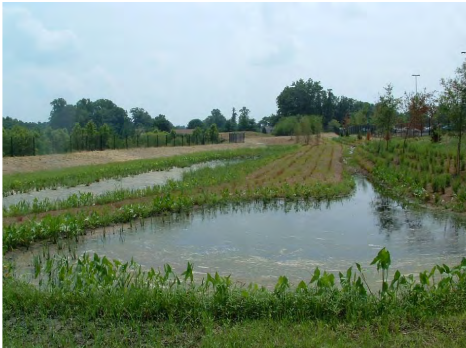
Wet Pond Facility Example
