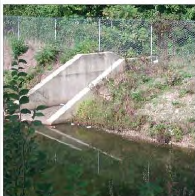
Do not suspend fence over outfall openings as shown above. (See photo to right)
