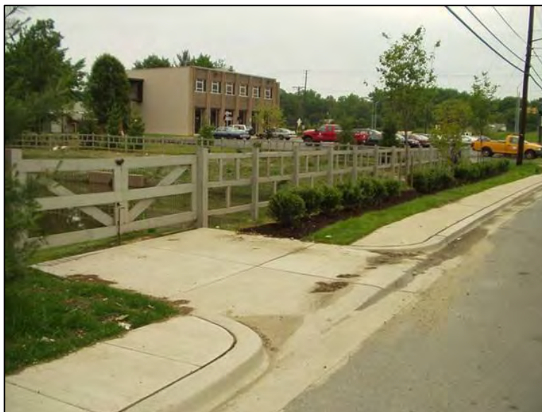
Figure 6-6. Concrete Apron and Depressed Curb Provided at Maintenance Access
