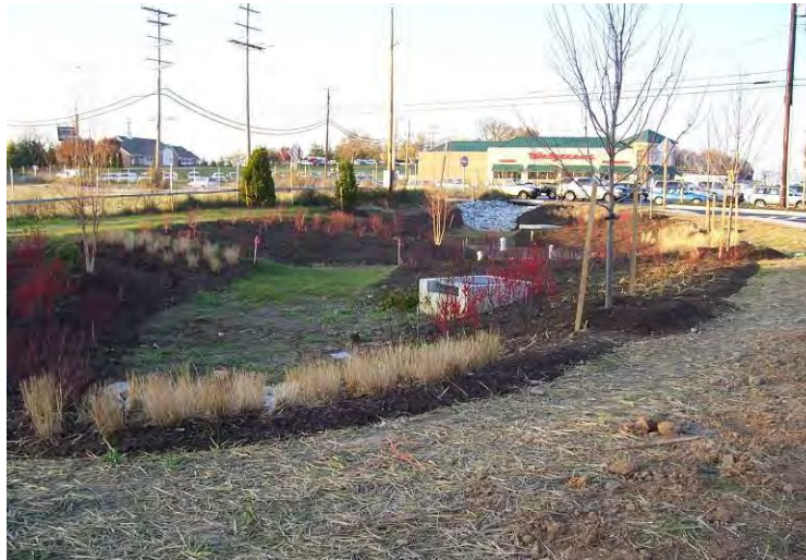
Sand Filter Facility Example
