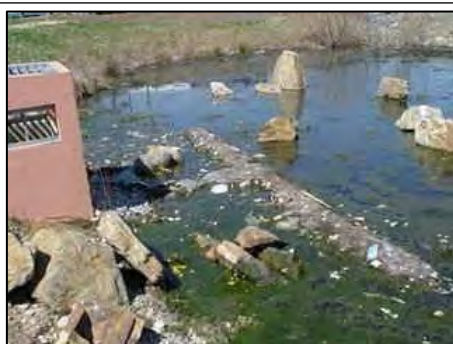
Low Flow Device uses a T-Connection and Runs Parallel to the Side Slopes (Preferred)
