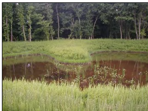
Baffle Constructed In-Situ Holds Form Over Time
