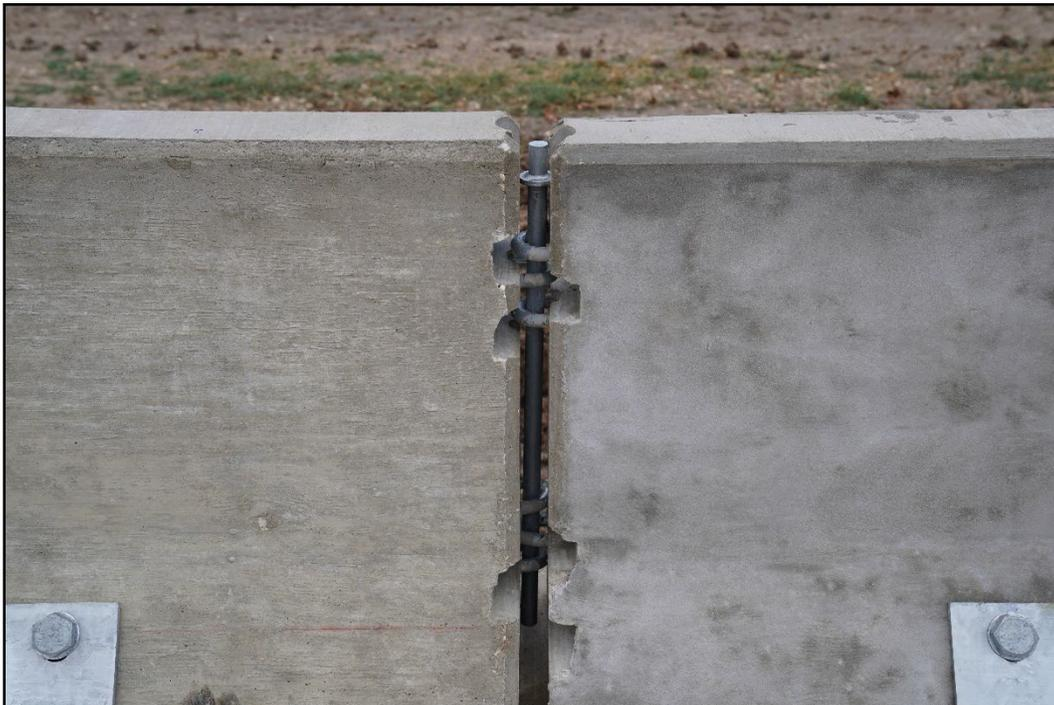
**Figure 3.7. Maryland F-Type Temporary Barrier prior to Testing—Segment Connection Details.**
