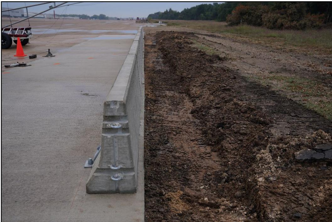
**Figure 3.3. Maryland F-Type Temporary Barrier prior to Testing—Back View of the Installation.**
