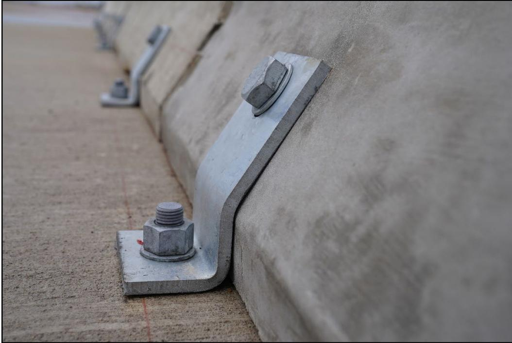
**Figure 3.6. Maryland F-Type Temporary Barrier prior to Testing—Ground Connection Details.**
