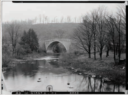
Casselman River Bridge, Grantsville, Garrett County Maryland
