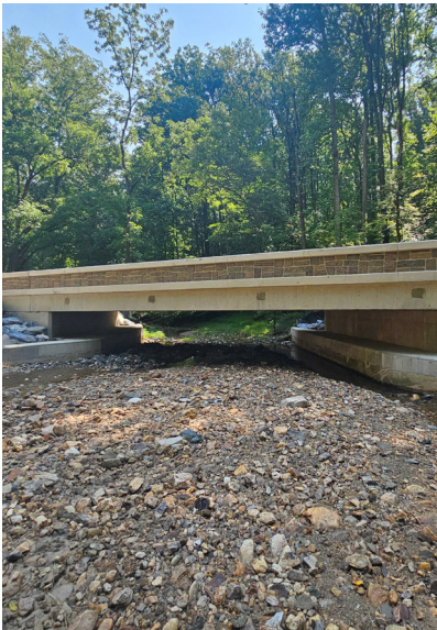
Henryton Road Bridge Howard County
