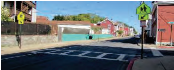
There is an uncontrolled marked crosswalk across Locust Street at Ray Street.
