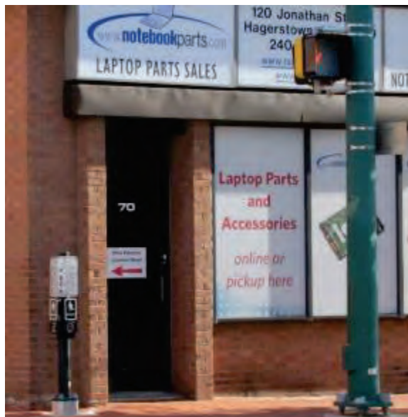
The pedestrian push buttons at Franklin Street and Jonathan Street are co-located and do not have an audible notification to pedestrians.
