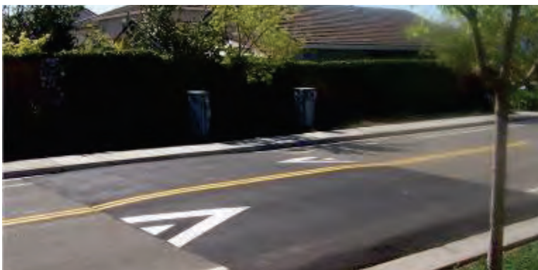
Speed hump at a residential street makes drivers to reduce their speed (Photo: NACTO).
