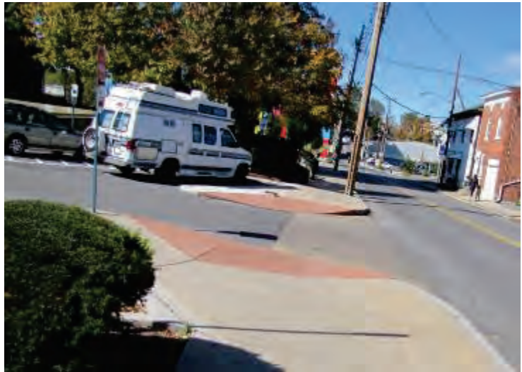
A driveway crossings connect sidewalks at a parking lot entrance in Hagerstown.
