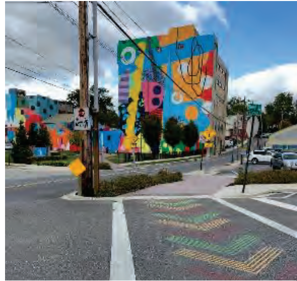
High-visibility crosswalk is painted in different colors at Hood Street and West Baltimore Street.
