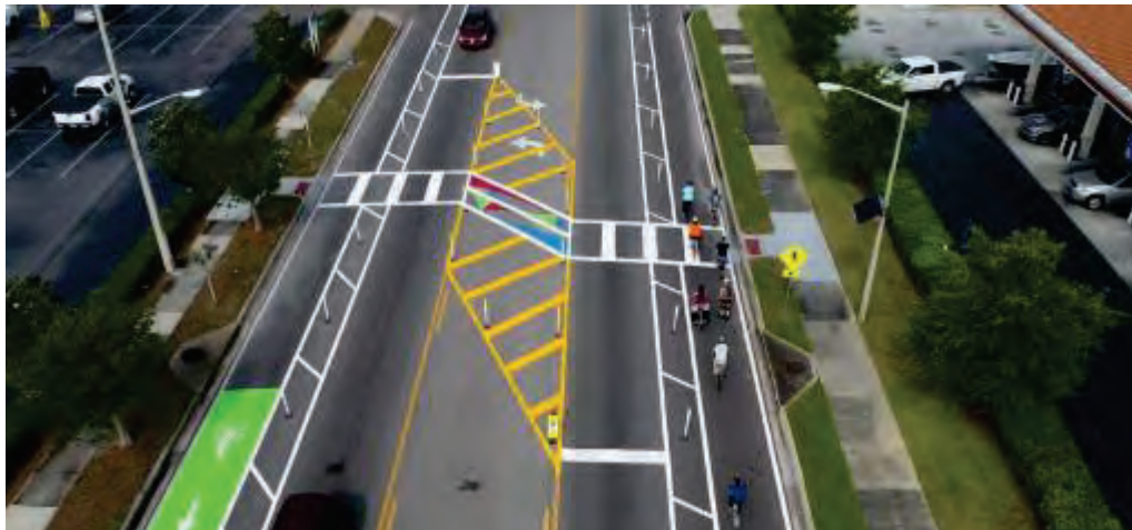
Demonstration of Curry Ford Road Diet including protected bike lane at each direction and a crosswalk with high visibility in Orlando, FL (Photo: bungalow.com).
