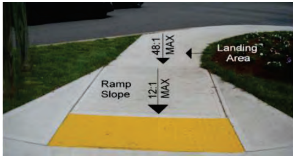
Maryland standard ramp 655.11 connects a corner of sidewalk to ADA area.
