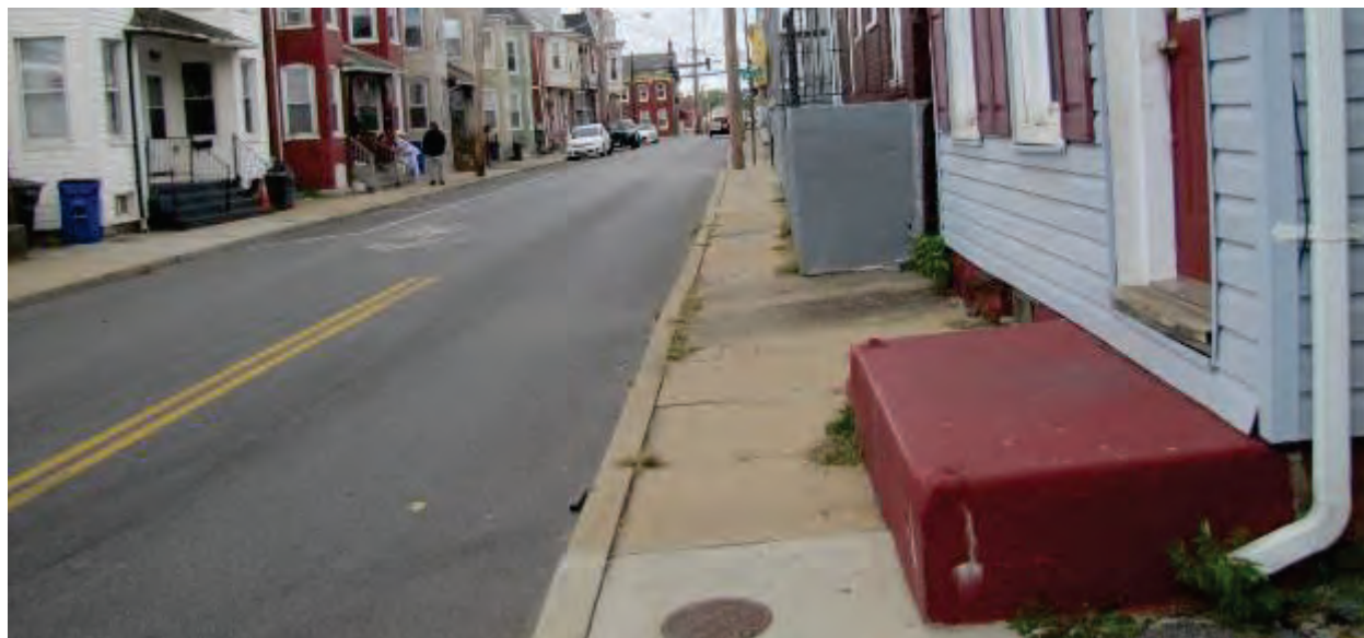
Residential stoops encroach on the sidewalk, narrowing space for pedestrians (Lee Street between Locust Street and Potomac Street).
