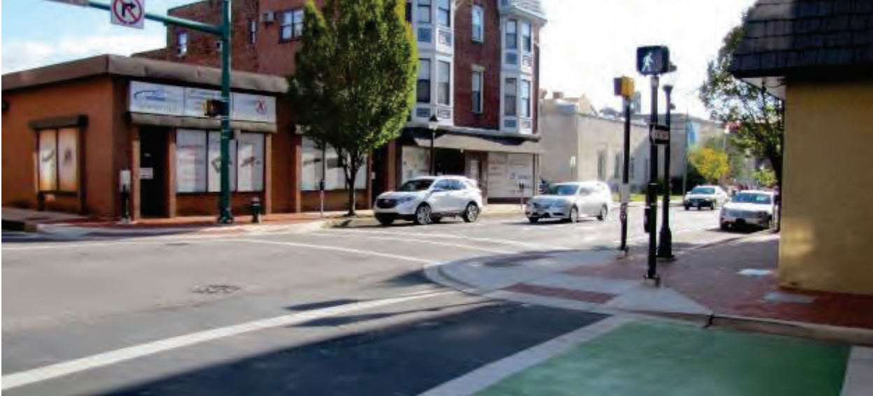
Pedestrian Signal at West Franklin Street provides pedestrians with crossing time.
