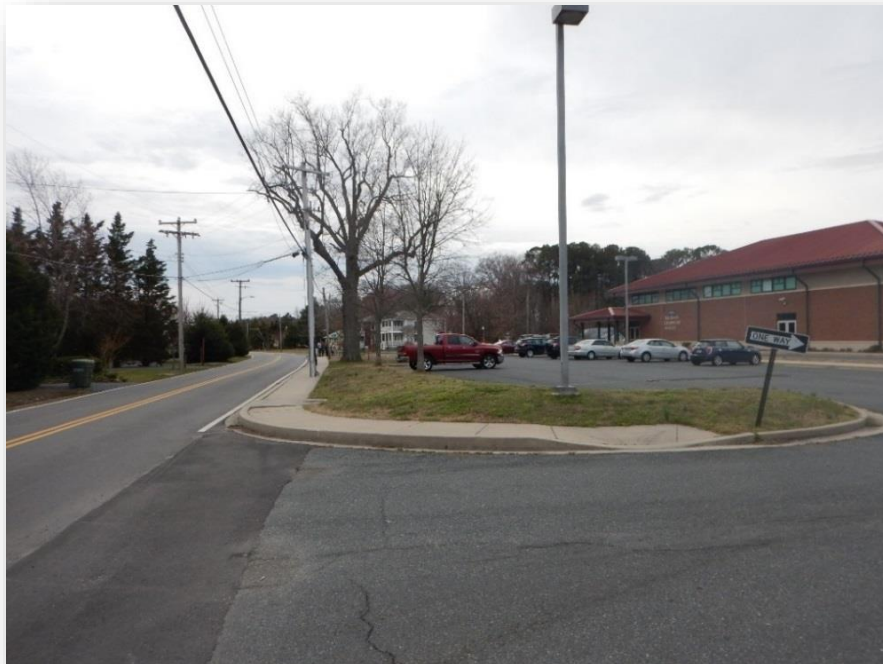
Figure 8 – Existing Concrete Sidewalk at Tilghman Elementary School (Looking south)
