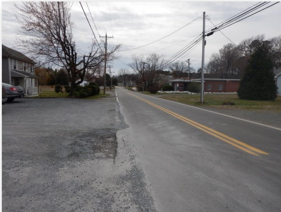
Figure 9 – Existing Utility Poles Along Both Sides of MD 33 (Looking south from Gibsontown Road)
