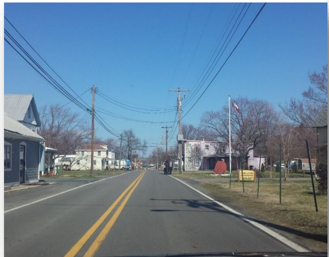
Figure 1 – MD 33 (Tilghman Island Road)
