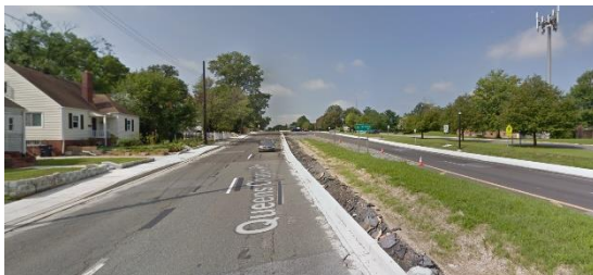
MD 500 @ MD 410: Northbound Lane – South view
