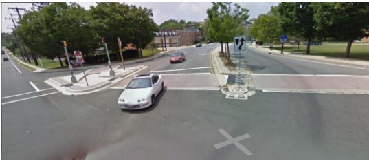
Belcrest Road @ MD 500: Southbound Lane – North view
