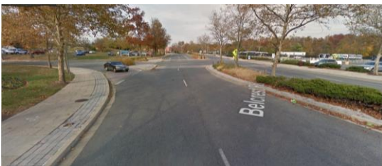
Belcrest Road @ Toledo Terrace: Southbound Lane – North view
