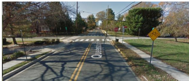
Queensbury Road @ 41 st Avenue: East view
