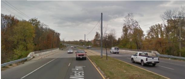
Westbound Lane – East view
