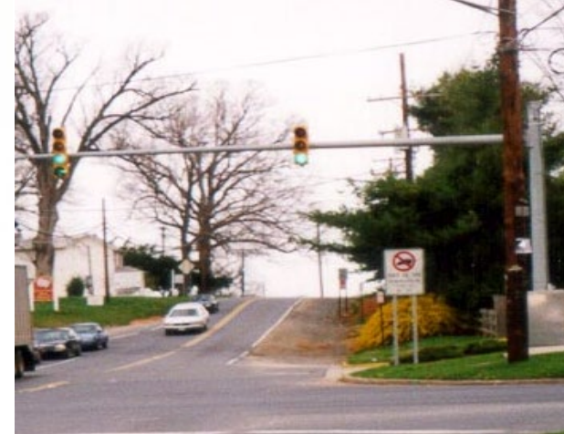
Temporary Traffic Signal
