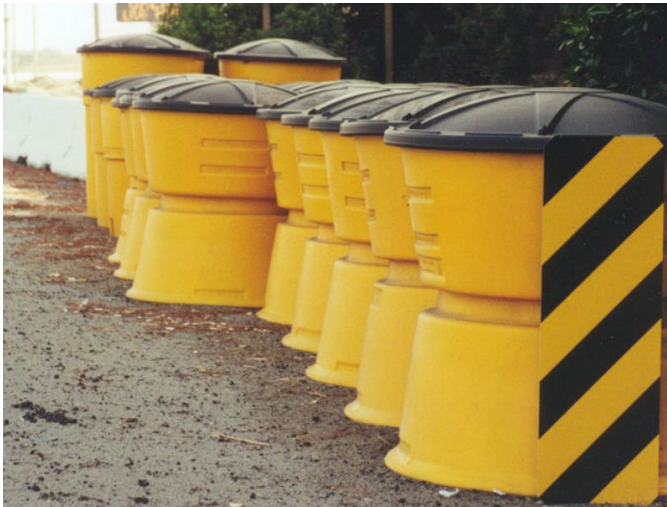
Non-re-directive Sand-Filled Plastic Barrels
