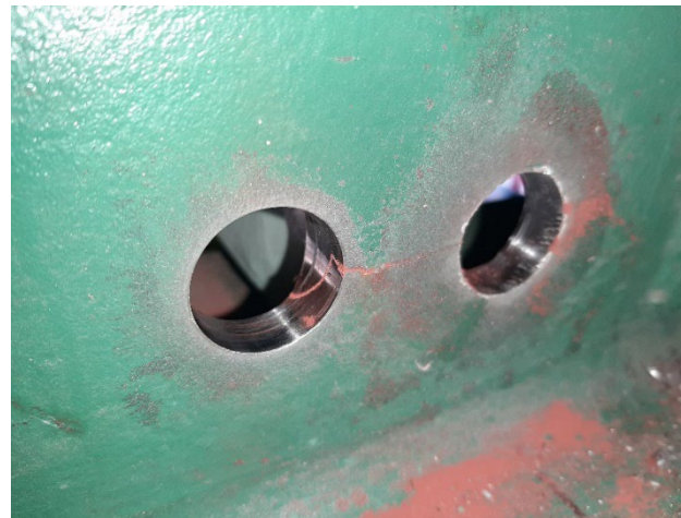
I-495 over Good Luck Rd. Crack Arrest
