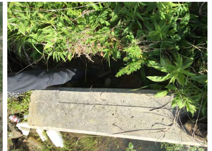
Minor Erosion Behind End Structure
