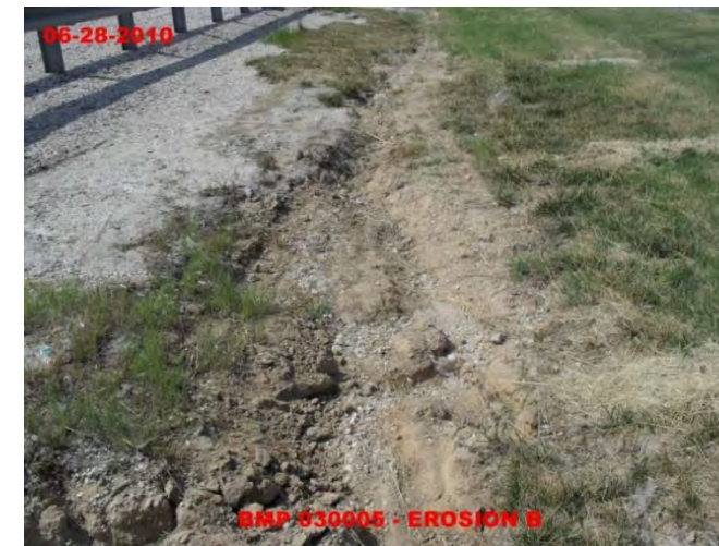
Minor Erosion in Grass Swale
