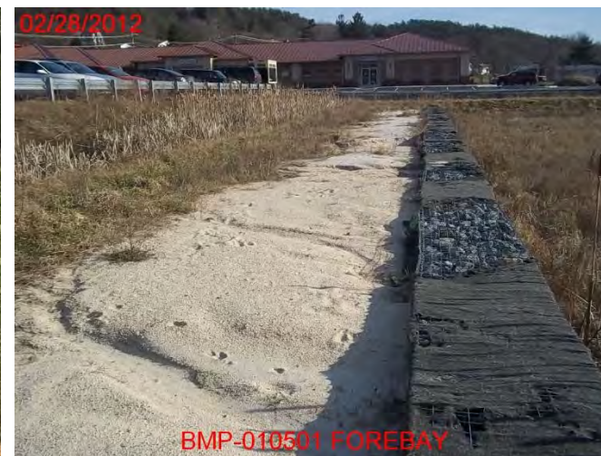
Major Sediment Accumulation in Forebay
