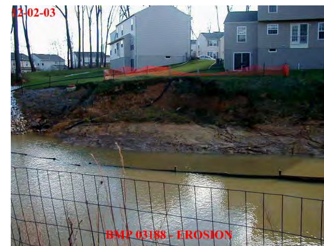
Major Erosion Along Pond Bank
