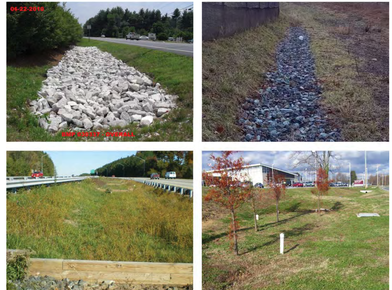
SAMPLE INFILTRATION FACILITY PHOTOS
