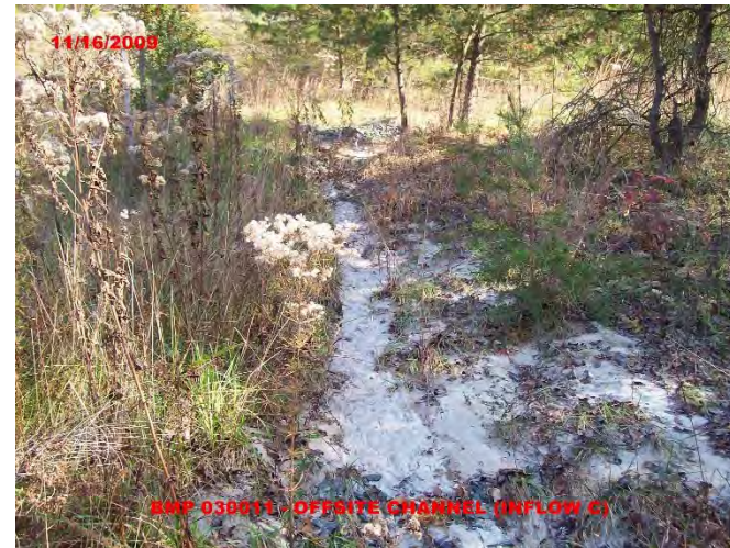
Minor Sediment Accumulation in Inflow Ditch
