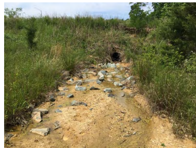
Major Sediment Accumulation at Outfall
