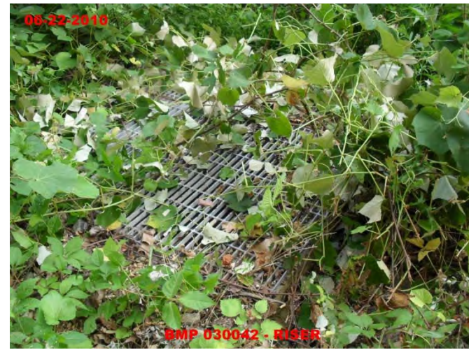
Vegetation Obstructing Outflow Point
