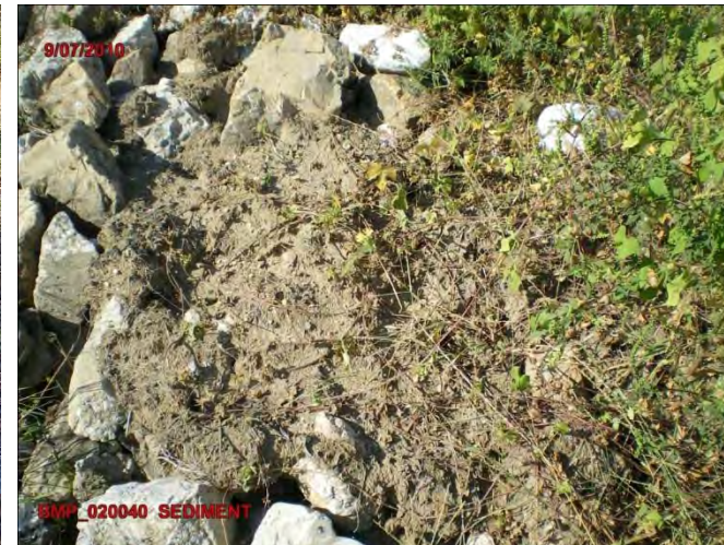
Minor Sediment Accumulation
