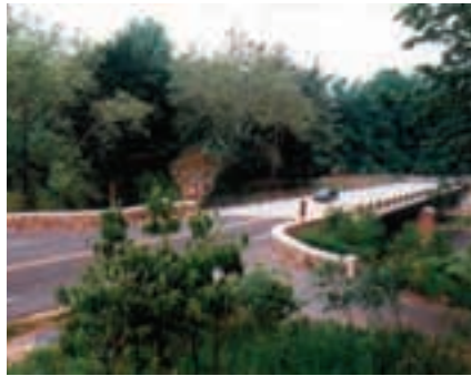
Open rail system is used on MD 161 over Deer Creek to retain open views.
