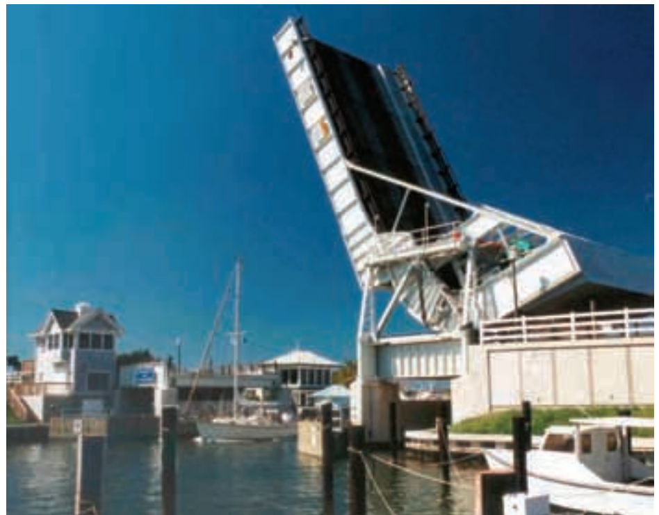
The bottom image shows the new bridge as it is today. The old bridge has been moved to the grounds of a local museum.
