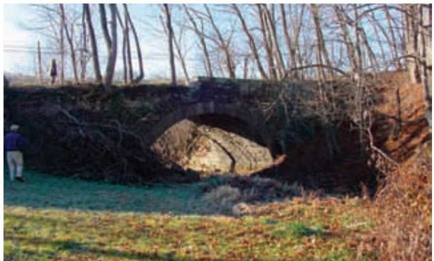
Preservation or stabilization of these stone arch bridges along old alignment over Big Shade Run is desperately needed.
