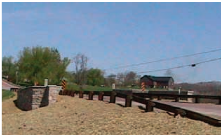
Creative use of steel backed timber rail to protect the bridge parapet wall on the Meadow Run Bridge help to retain the existing width of the historic bridge (photo by K.C. Keith, Maryland SHA)
