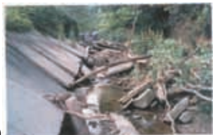
Soil bio-engineering concepts were used by Maryland State Highway Administration and Maryland Department of Natural Resources to restore Porter Run adjacent to the Historic National Road near Clarysville. Willow whips were interplanted to help stabilize the streambank. (photographs by SHA)
