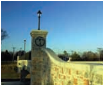
Context sensitive approach is used for new bridge for Dulaney Valley Road over I-695.
