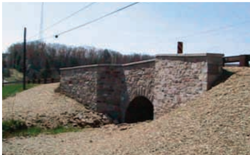
Recently reconstructed bridge over Meadow Run illustrates how small structures similar in scale and proportion to the old structures can be done. The stipulations in the Memorandum of Agreement between SHA and the Maryland SHPO (see sidebar, page 29) were simple and straight forward (photo by K.C. Keith, Maryland SHA)
