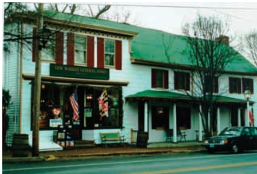
Within city and town streetscape efforts, decorative "acorn" fixtures have been installed as part of streetscape improvements in Frostburg (top) and colonial fixtures in New Market (bottom).
