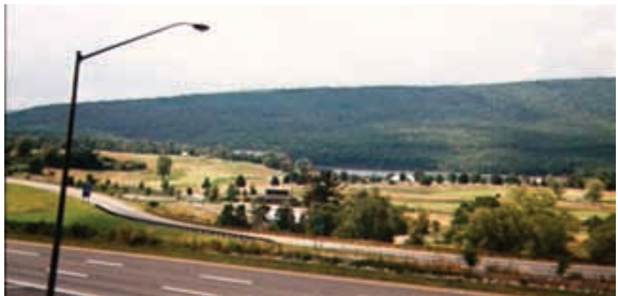
W-Beam with steel or wood post, weathering steel finish was installed along I-68 and rebuilt sections of Maryland 144 as shown near Rocky Gap resort (photograph by Richard Langton).
