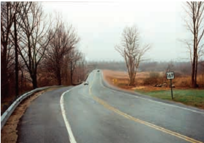
Simulation (below) illustrates potential impact of straitening out a curve on Route 169 (existing condition above). The simulation illustrates an increase in design speed of approximately 10 mph requiring longer sight lines, and removing more roadside vegetation. The result is an overall loss of scenic quality and a greater difference in operating speeds between leisure travelers and commuters.
