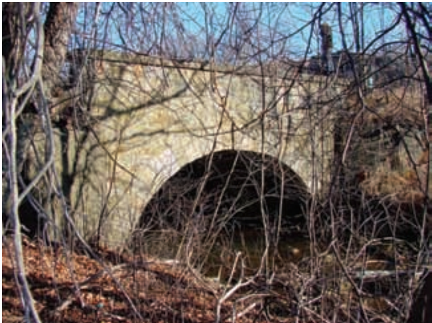
Remnant small structure over Big Shade Run (photo courtesy of Terry Maxwell, State Highway Administration)
