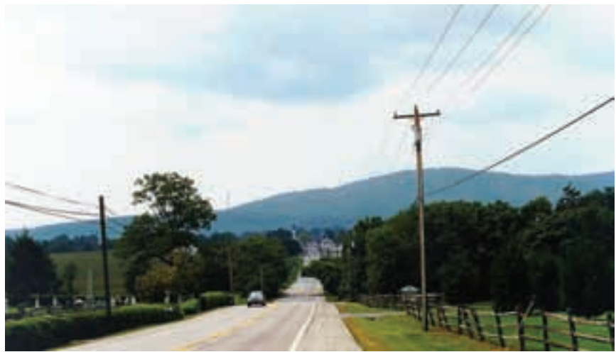
Participation by adjacent owners in maintenance of right-of-way is one strategy that should be encouraged along the Historic National Road (approaching Clear Spring, for example).
