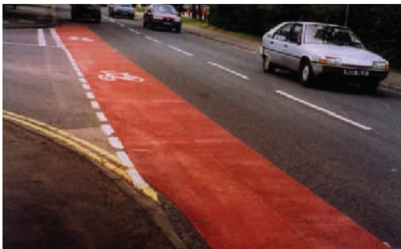
Example of modified epoxy binder application in Great Britain (photo courtesy of Jarvis-USA) preferred for bicycle use over chip seal.
