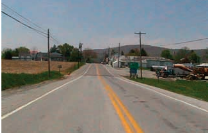
Historic National Road near Cool Hollow Road illustrates the current use of a wide edgeline treatment to help guide drivers around the sharp curve.
