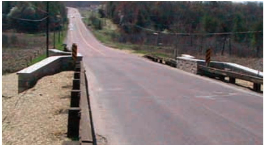
Steel-backed Timber Guardrail with dark brown stain was recently installed along the National Road approaching the Meadow Run Bridge (photograph by K.C. Keith, SHA).
