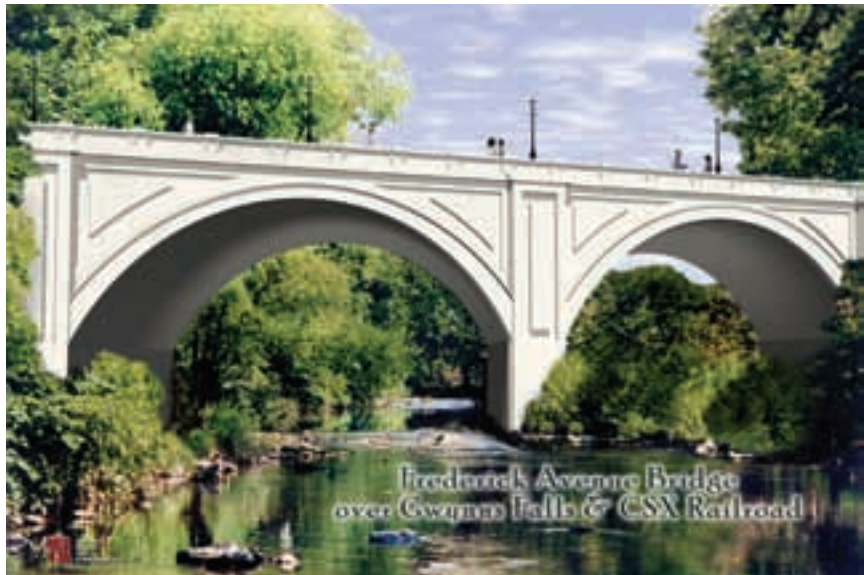
Gwynn’s Falls Bridge is slated for reconstruction by the City of Baltimore. The proposed preliminary design concept maintains the character-defining features of the bridge (courtesy of Whitney, Bailey, Cox and Magnini).
