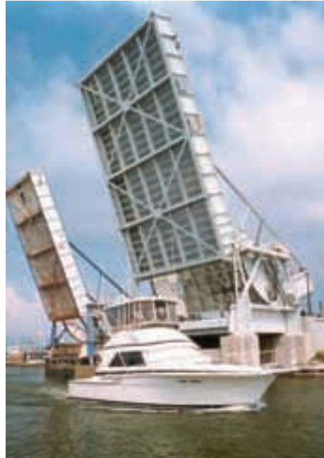
The new Knapps Narrows bridge (foreground) retains much of the look of its predecessor (background).
