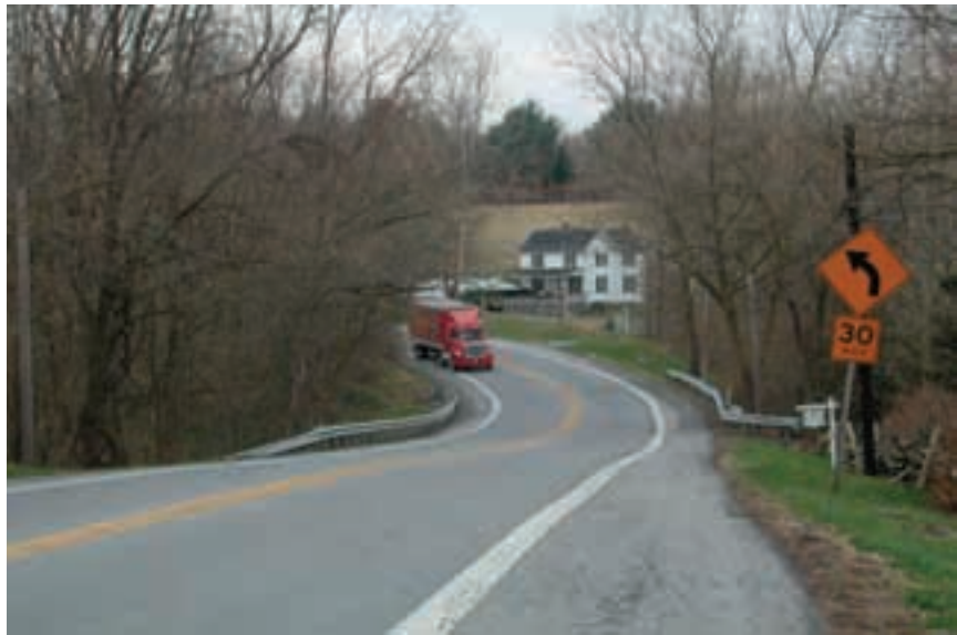
Historic National Road near Cool Hollow Road illustrates the current use of a wide edgeline treatment to help guide drivers around the sharp curve.
