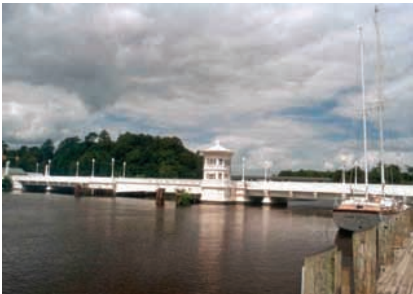
Reconstructed Pocomoke River bridge matches what previously existed, and was able to strengthen moveable portion of existing bridge so that it could remain.
