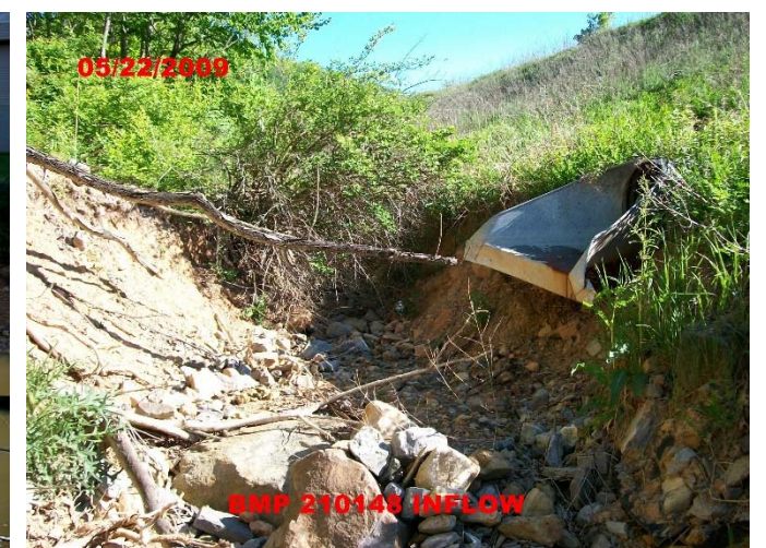
Major Erosion at Inflow Point
