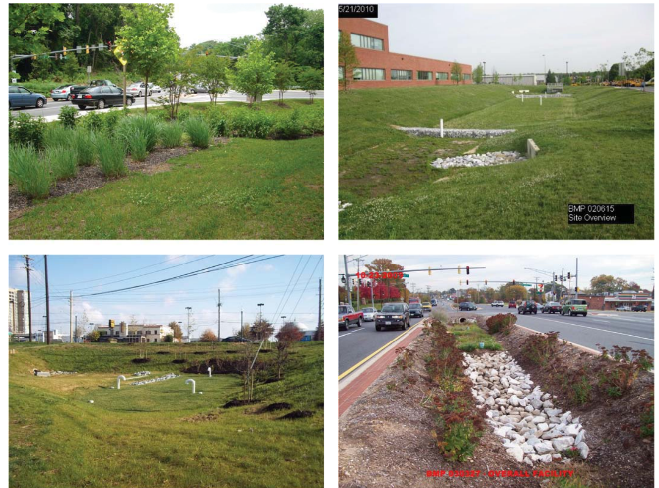
SAMPLE FILTRATION FACILITY PHOTOS
