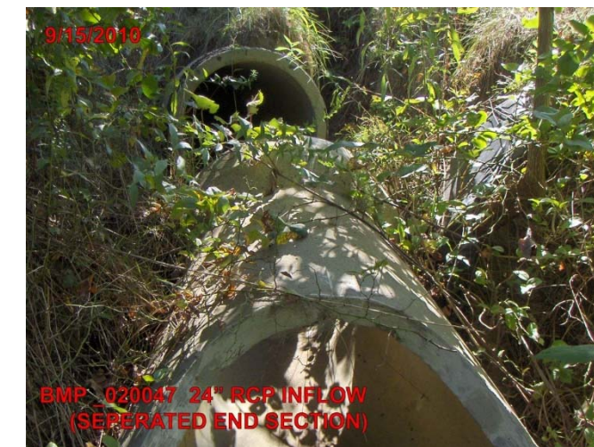
Pipe Separated From End Structure
