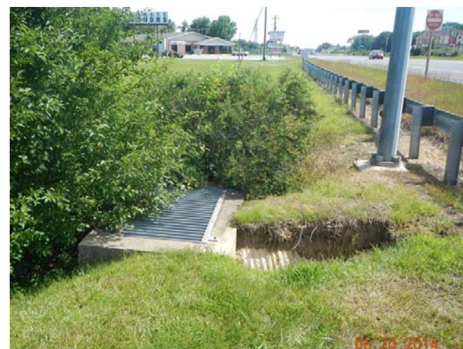
Eroded Embankment Exposing Pipe
