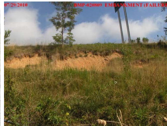
Eroded Embankment
