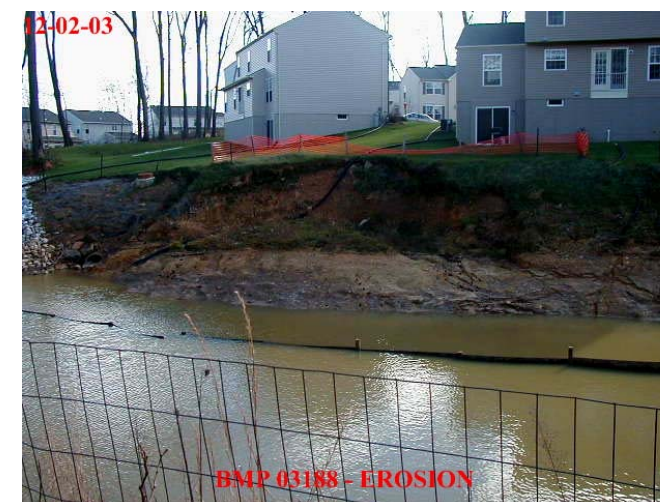
Major Erosion Along Pond Bank
