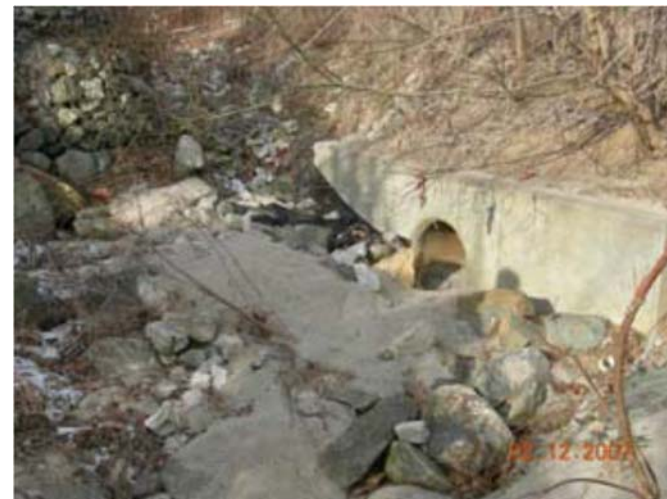
Major Sediment Accumulation at Outfall
