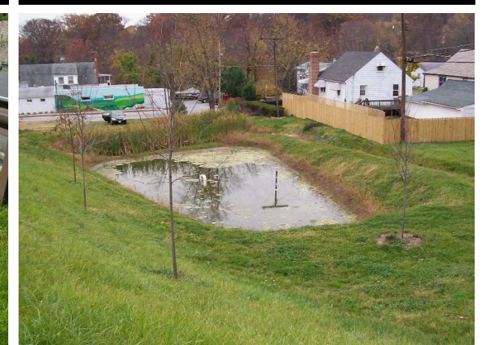
Surface Sand Filter Not Draining
