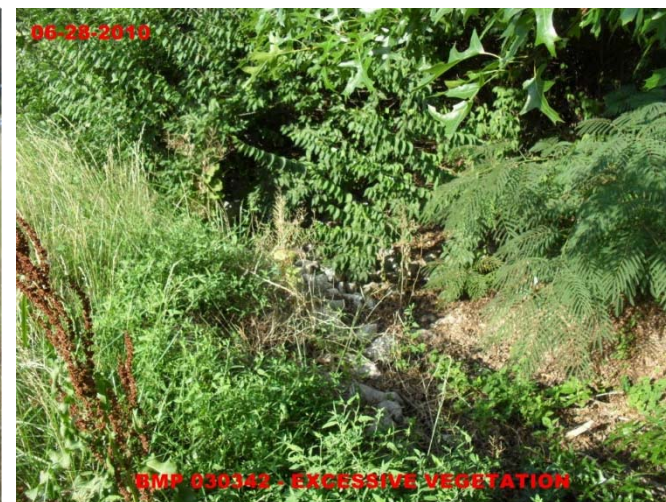
Excessive Vegetation in Infiltration Trench
