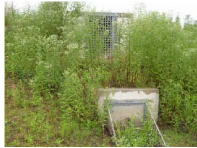
Vegetation Obstructing Riser Structure
