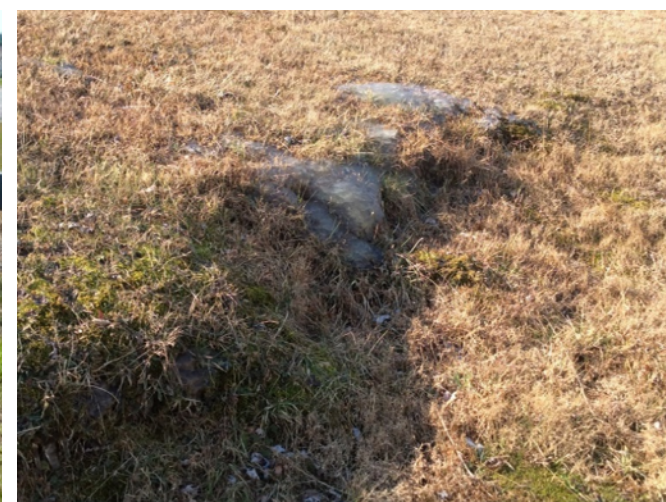
Frozen Seepage Through Embankment
