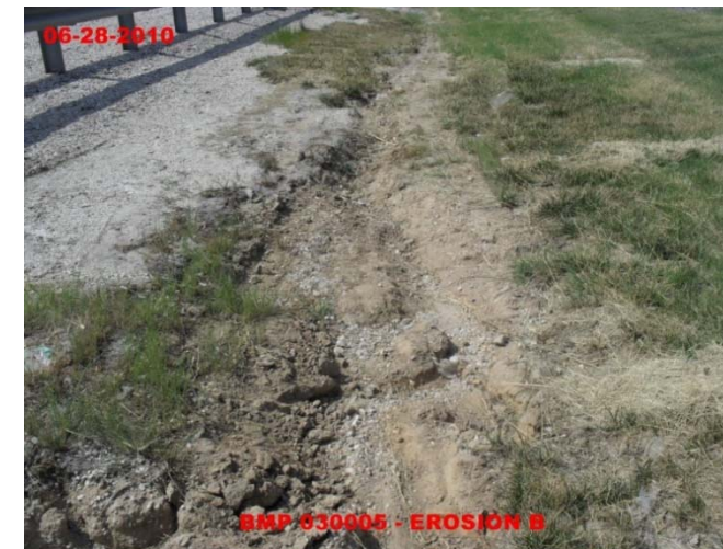
Minor Erosion in Grass Swale
