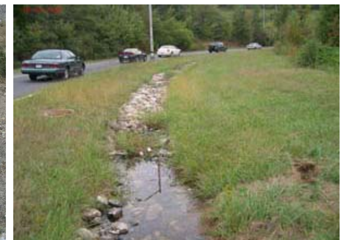
Saturated Infiltration Trench
