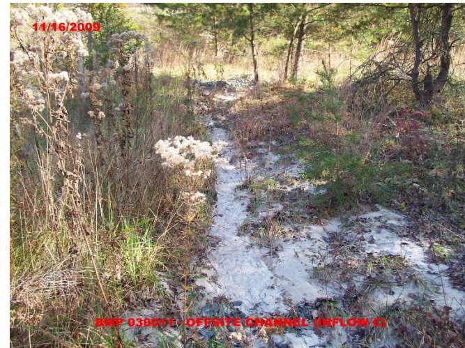
Minor Sediment Accumulation in Inflow Ditch
