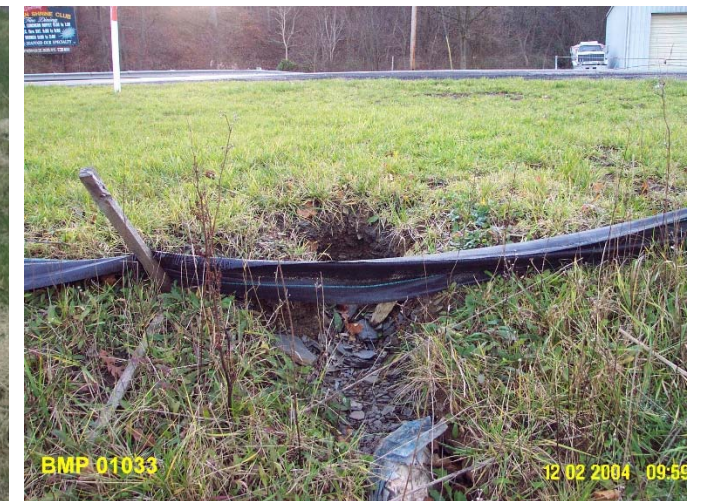
Minor Erosion Under Silt Fence
