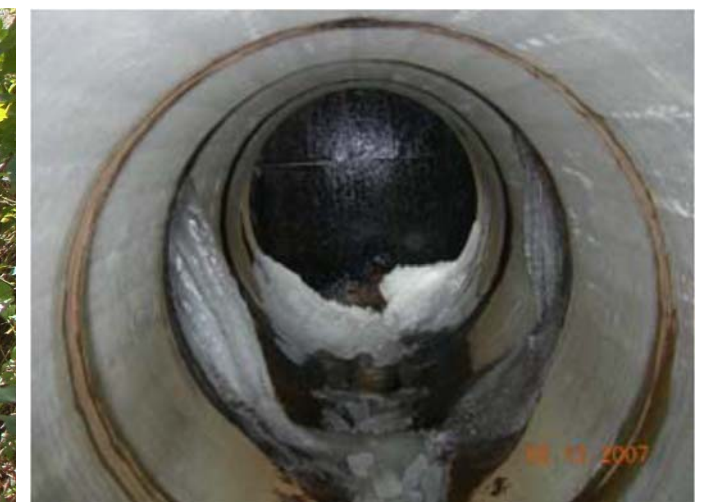
Water Leaking into Pipe
