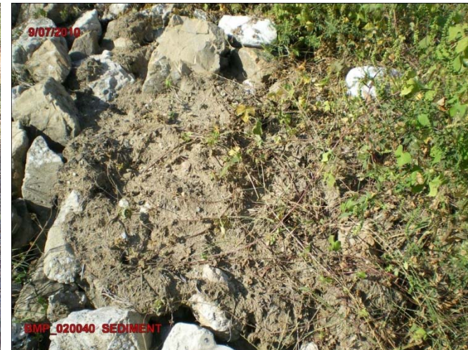
Minor Sediment Accumulation
