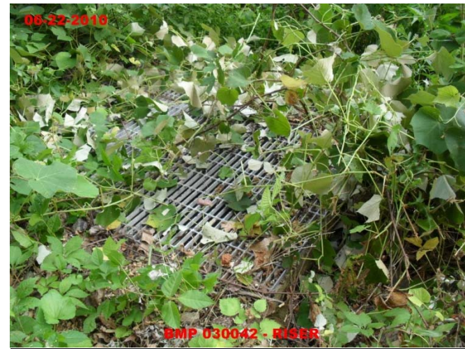
Vegetation Obstructing Outflow Point
