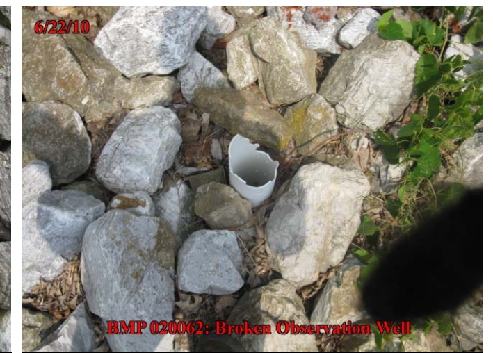
Broken Observation Well
