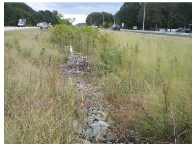
Excessive Vegetation in Infiltration Trench
