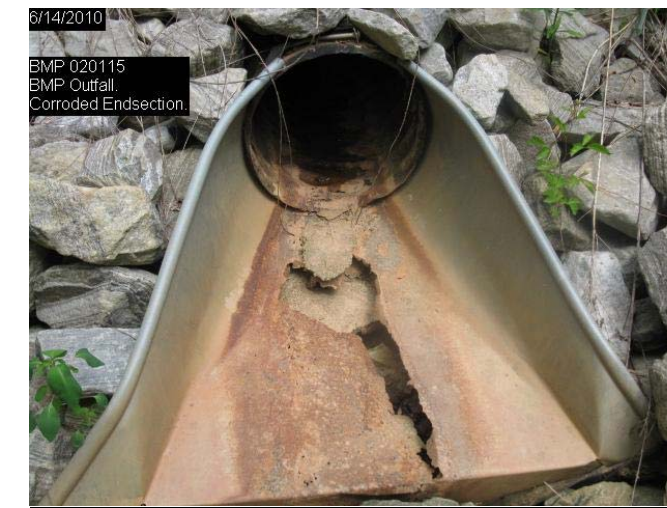
Deteriorated CMP End Structure
