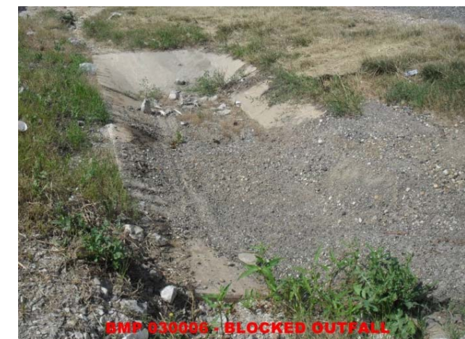
Accumulated Sediment Blocking Outfall Point
