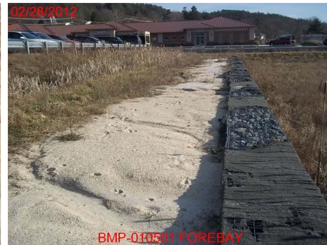
Major Sediment Accumulation in Forebay
