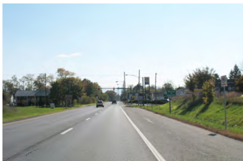
Figure 13 Entering Hagerstown from the west
