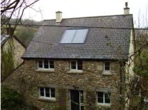
Figure 76 Solar panels integrated sited on historic structure to minimize impact, Dartmoor, UK
