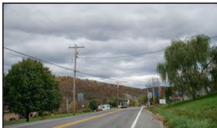
View southeast entering Flintstone from the west on MD 144
