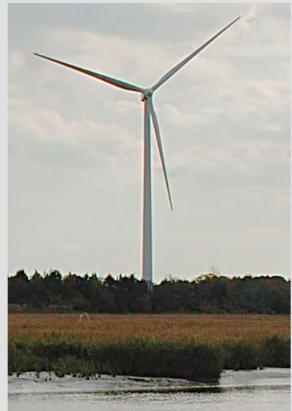
Figure 74 Wind turbines are often 400' tall to the blade tip
