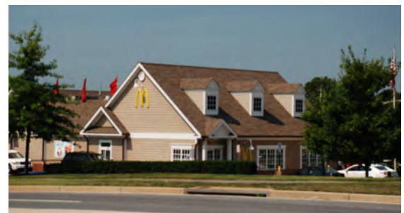
Figure 61 McDonalds in Urbana, MD adapted it's architectural style to the desired character of the community
