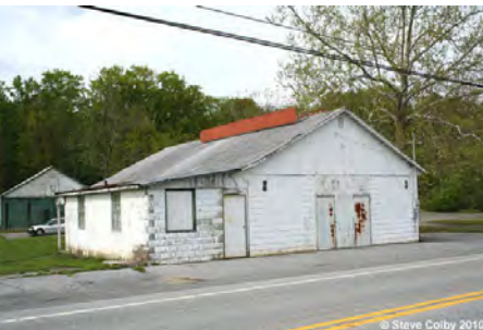
Figure 37 Big Pool Garage (photo courtesy of Steve Colby)
