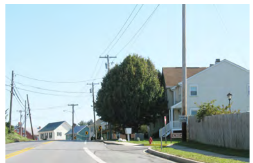
Figure 16 New townhouses in Middletown complement surrounding structures.
