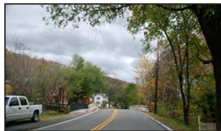
View southeast crossing Flintstone Creek on MD 144 traveling eastbound
