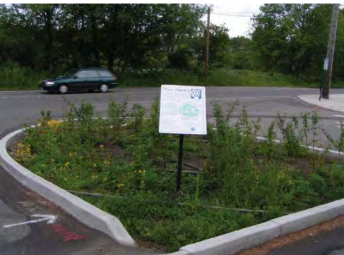
Figure 59 Infiltration area incorporated into Howard County's Government Center parking lot
