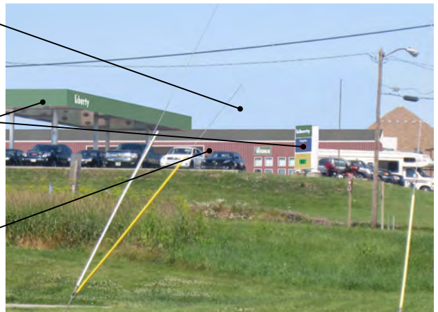
View A. Example of renovations to existing stand alone commercial to use as guidelines for future development.
