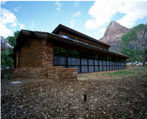
Figure 75 Solar panels integrated directly into the design of the visitor center at Zion National Park, Utah as part of new construction
