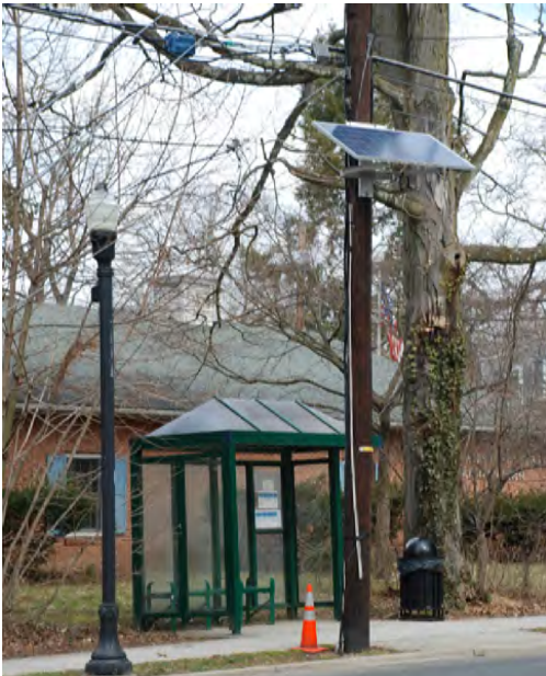
Figure 73 Distributed solar PV panel is linked to a network of panels along existing utility poles in Lawrenceville, NJ. The cumulative impact of these distributed arrays, when placed on every utility pole with solar access is significant
