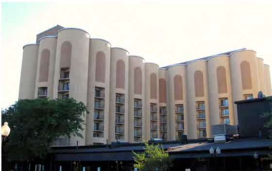
Example of adaptive reuse at the Quaker Square Inn, Akron, OH
