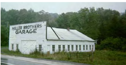
Figure 36 Former Miller Brothers Garage, Allegany County
