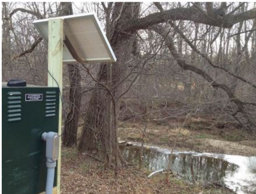
Figure 8. U.S. Geological Survey downstream station (Site ID 01636846) on Little Catoctin Creek near Rosemont, MD.
