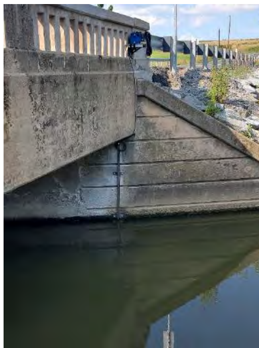
Figure 5. FY23 upstream station (Site ID 01636845) on Little Catoclin Creek near Rosemont, MD. The photo shows the ISCO velocity and area flow module.
