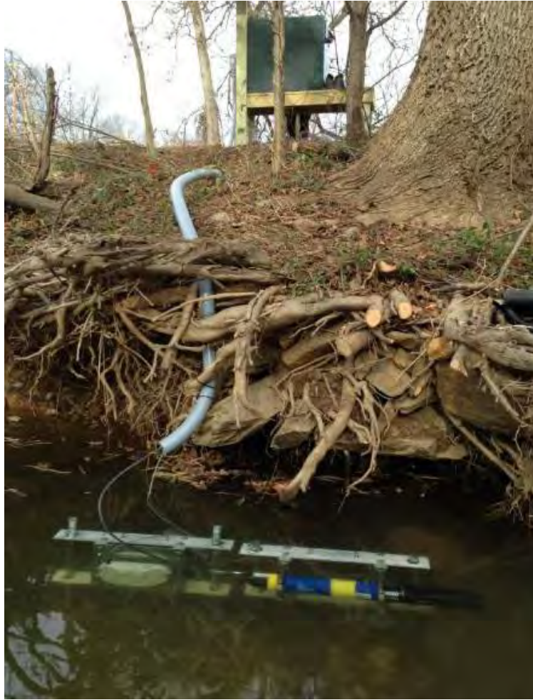
Figure 9. U.S. Geological Survey the downstream station (Site ID 01636846) on Little Catoctin Creek near Rosemont, MD. The photo shows the temporary gage station and the discharge and water-quality sonde installed in the river.
