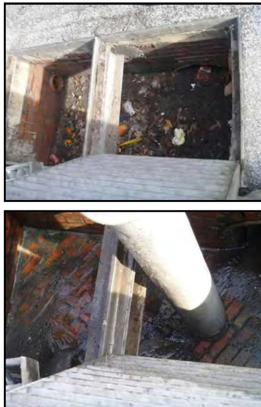
Figure 10: Inlet Before and After Cleaning
