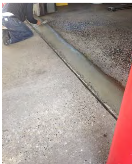
Figure 4: Wash Water Berm Install
