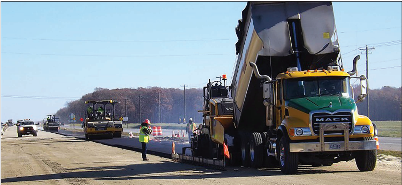
Progress on MD 404 near Church Lane.
