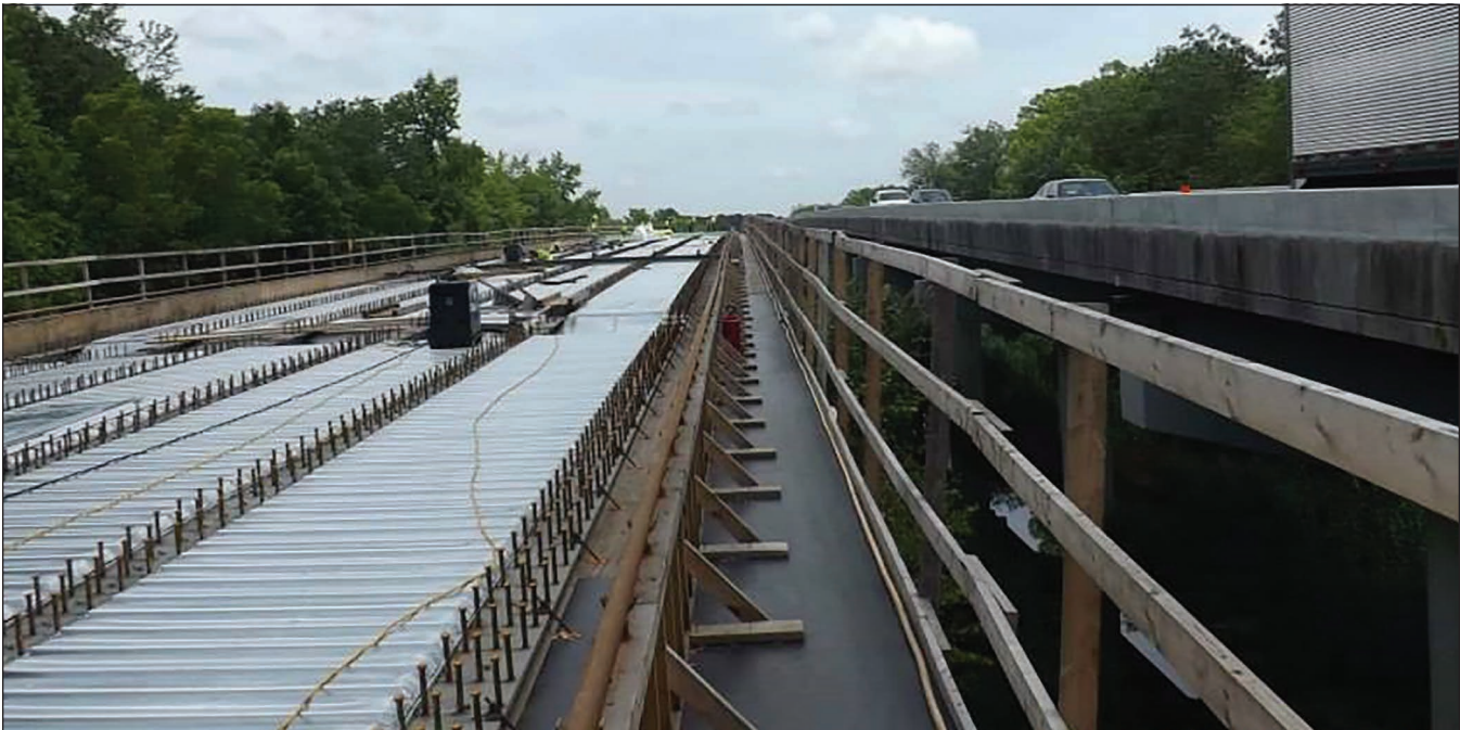
Southbound US 13 bridge.
