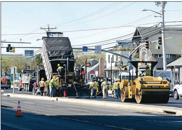
Coastal Highway (MD 528) resurfacing.
