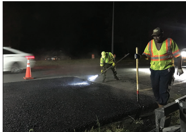
I-495 resurfacing in Montgomery County.
