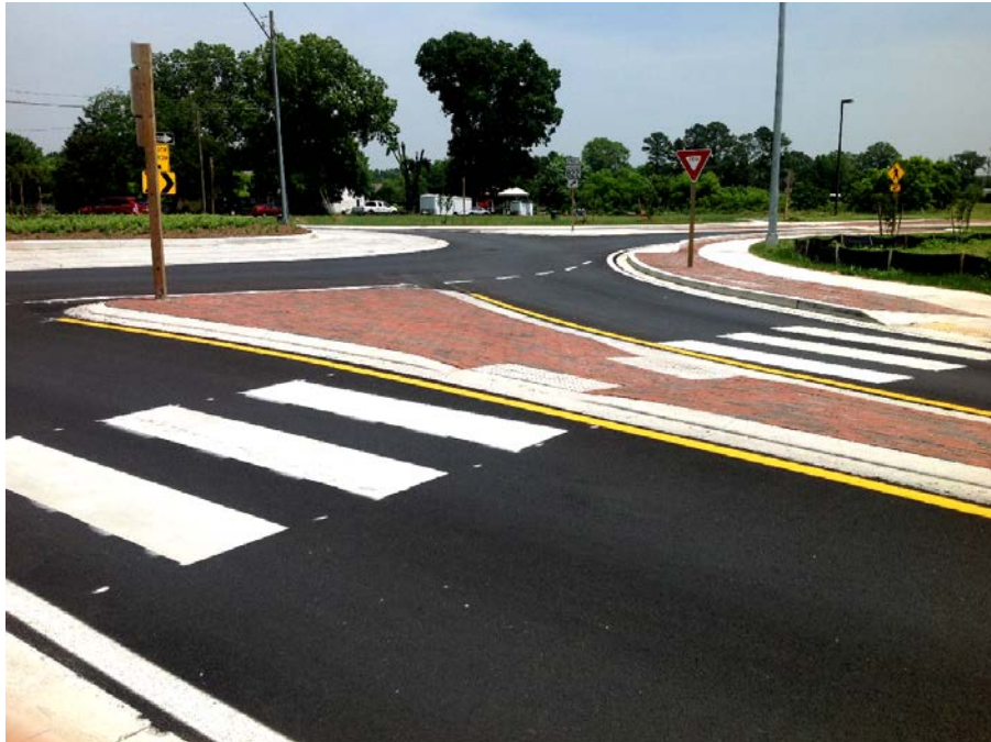
(SHA Photo: Completed Traffic Circle (Roundabout) on MD 675 (UMES Boulevard) Near the /University of Maryland Eastern Shore in Princess Anne, Maryland
