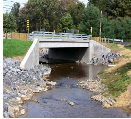
Completed US 219 Bridge, October 2014
