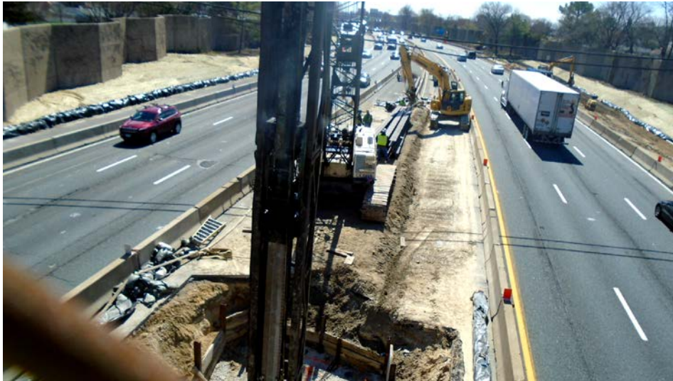
(SHA Photo: View from a crane on I-695 (Baltimore Beltway) between MD 41 (Perring Parkway) and MD 147 (Harford Road) - Widening/Interchange reconstruction) (Summer 2015)
