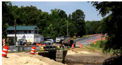
(SHA Photo: MD 5 Bridge over Eastern Branch Replacement Project - June 2015)
