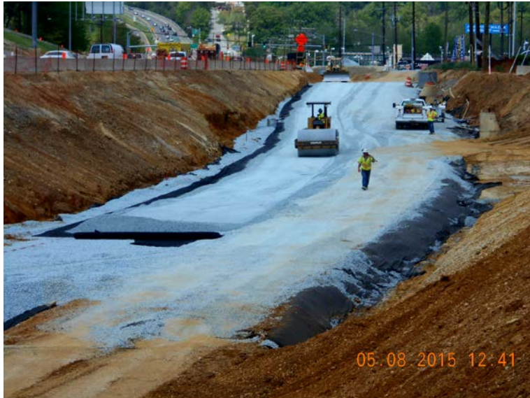
(SHA Photo: New northbound MD 5 alignment at Auth Way project in Camp Springs, May 2015)
