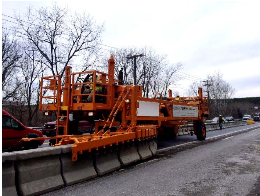
(SHA Photo: "The Zipper Machine" Moving Concrete Barriers to Accommodate Directional Traffic during Bridge Construction on the MD 140 Bridge over the Patapsco River - spring 2015)
