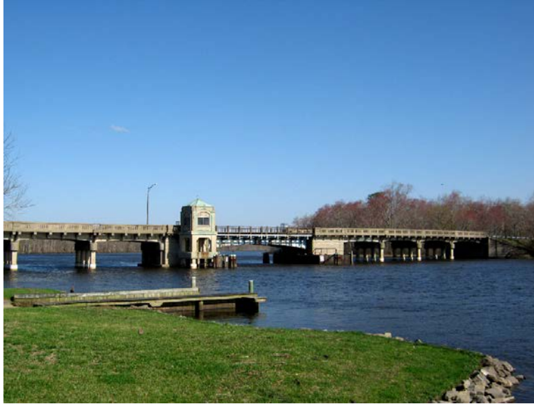
(SHA photo: MD 14 (Rhodesdale Eldorado Road) over Marshyhope Creek in Dorchester County.)
