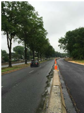
(SHA Photo: MD 22 near Aberdeen Proving Grounds Widening Project - spring 2015)
