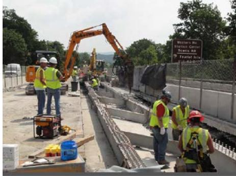
*SHA is replacing the deck (driving surface) for the I-68 bridges over Kelly Boulevard and Patterson Avenue in Cumberland. Here, crews are removing the deck on the central section of the Patterson Avenue Bridge.*
