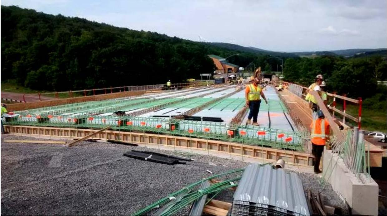
*(SHA photo: The MD 546 (Finzel Road) Bridge over I-68. Crews installing new bridge deck (driving surface. Bridge is now opened.)*
