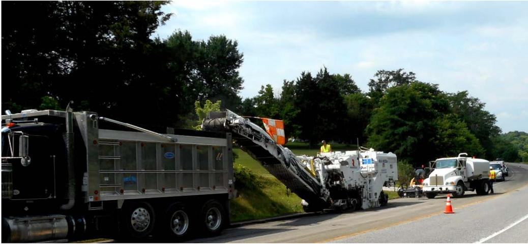
*(SHA photo: Crews milling (removing top layer of asphalt) on MD 34 (Shepherdstown Pike in Washington County.)*
