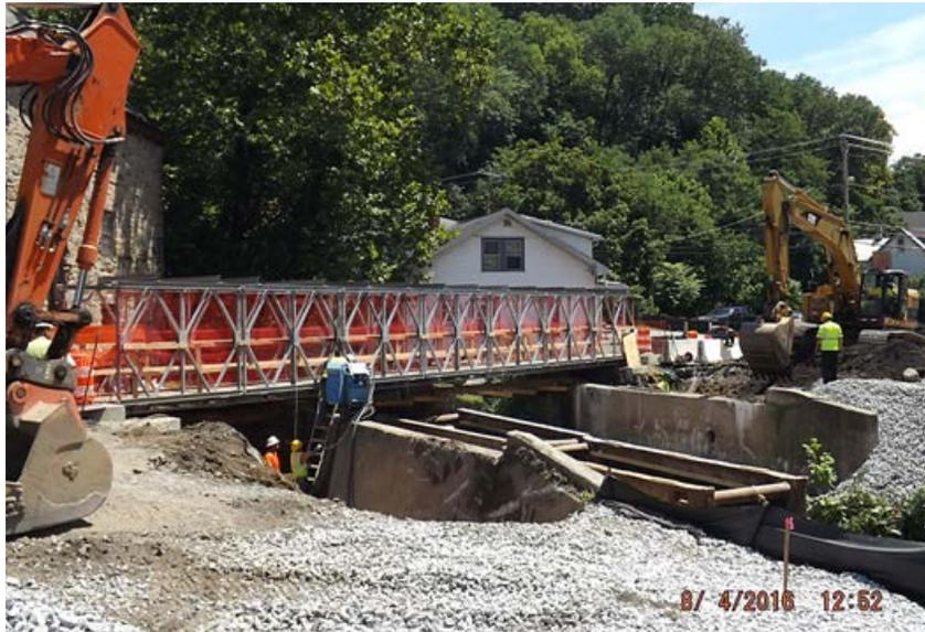
(SHA Photo: [MD 222 Bridge over Rock Run](#). Old bridge is gone and a temporary pedestrian walkway has been installed for access to local businesses. August 2016.)
