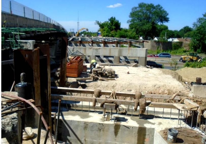
*(SHA Photo: Removing old steel beams and demolishing Old Harford Road Bridge over I-695. The new Old Harford Bridge over I-695 opened early-June 2016. This is part of the [I-695 between MD 41 \(Perring Parkway\) and MD 147 \(Harford Road\)-Widening/Interchange reconstruction](#))*
