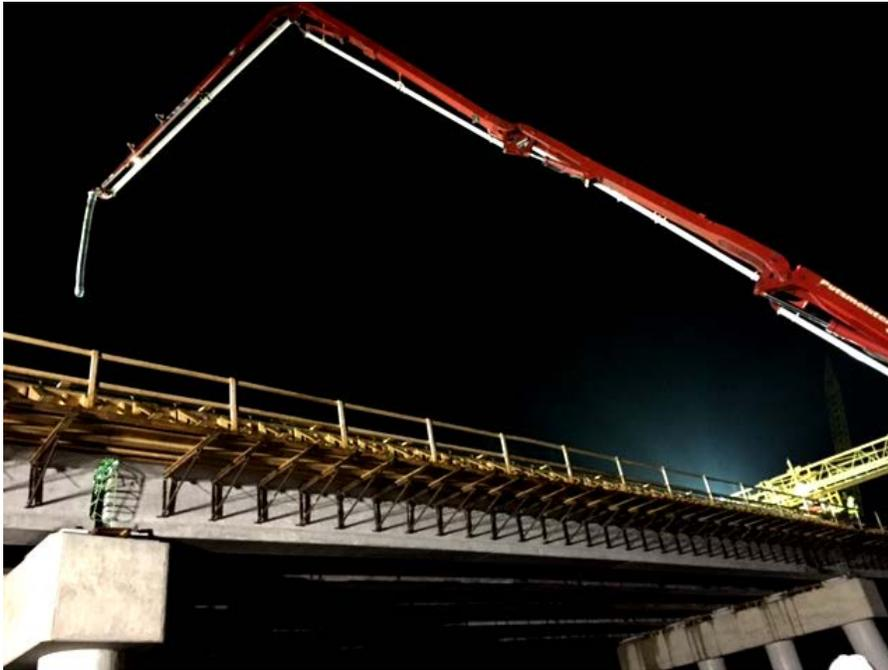
*(SHA Photo: Concrete bridge deck pour for the new Dover Bridge project ([MD 331 Bridge over Choptank River at the Caroline/Talbot County line.](#)) (August 2016)*
