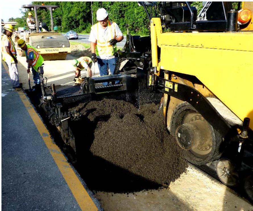
(SHA photo: Widening [northbound US 29](#) in Columbia is almost complete. Here, crews are using recycled pavement for the new lane.)
