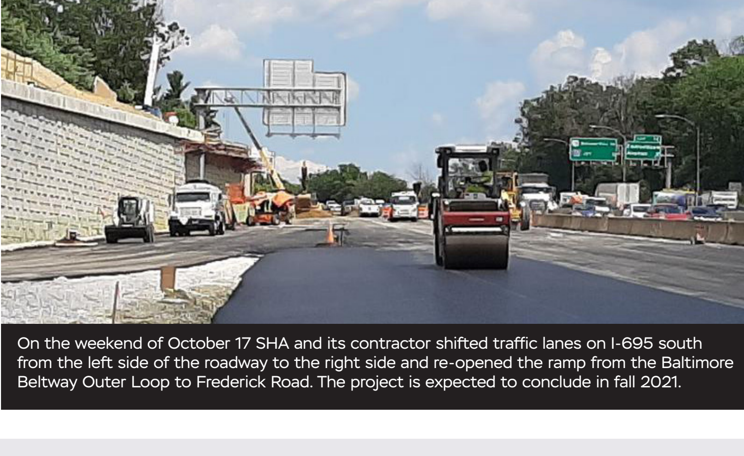
On the weekend of October 17 SHA and its contractor shifted traffic lanes on I-695 south from the left side of the roadway to the right side and re-opened the ramp from the Baltimore Beltway Outer Loop to Frederick Road. The project is expected to conclude in fall 2021.
