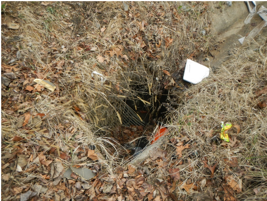
Inlet at STA 111+50 RT (just upstream of POI 4) – grate missing, will need to be replaced in both options
