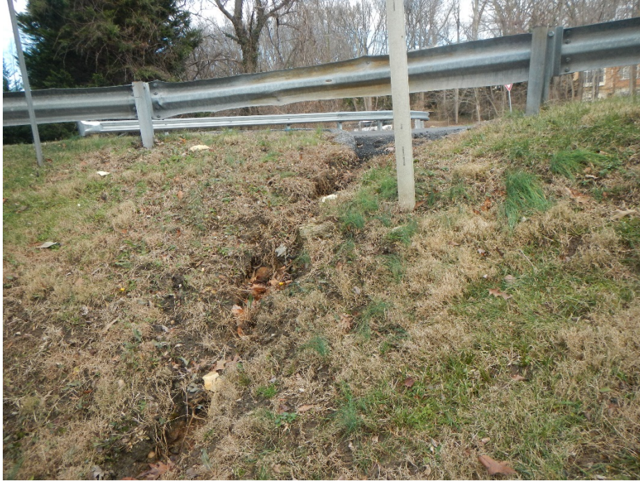
Erosion at STA 111+50 RT – will need to be stabilized
