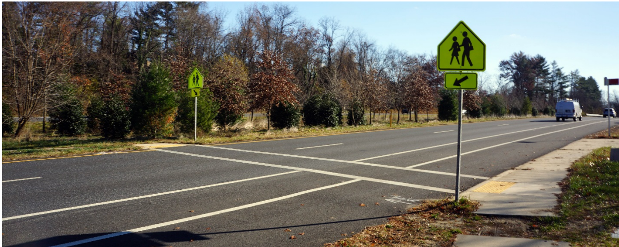
Figure 9: Pavement markings at the Pyle Road crosswalk are missing diagonal hatching
