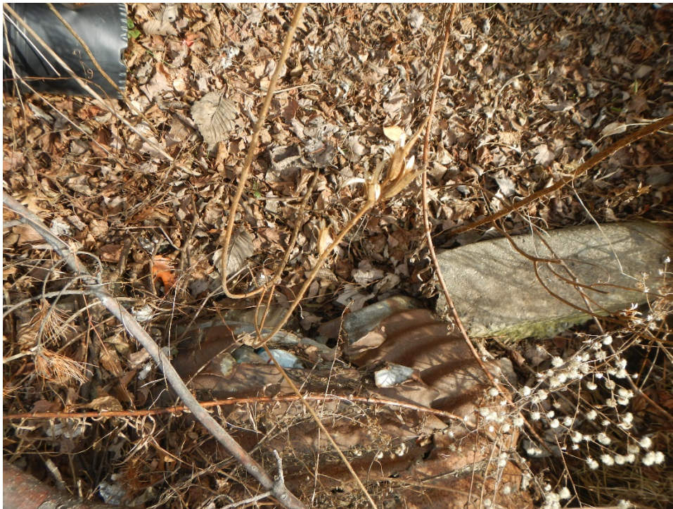
Outlet at STA 127+75 LT (upstream of POI 5)– end of pipe is crushed and will need to be replaced in both options.
