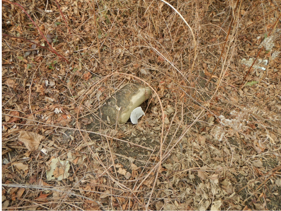
Existing outfall at STA. 123+30 in the median – 90% sedimented, will required pipe cleaning if option 2 is pursued.
