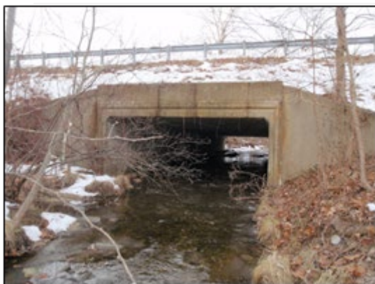
Example: Box Culvert
