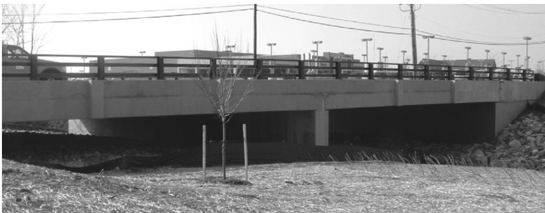
Figure 3.4. MD 7 over White Marsh Run (existing bridge).
