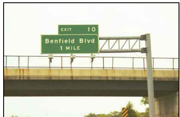
Figure 15 - Typical Plane Truss Cantilever
