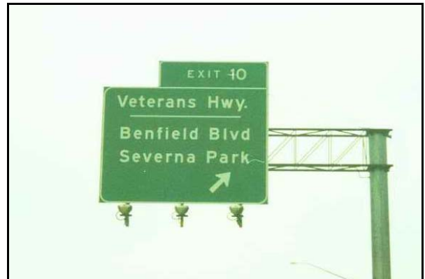
Figure 14 - Typical Box Truss Cantilever
