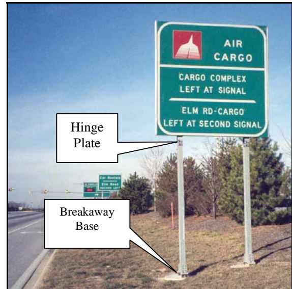
Figure 24 – Breakaway Steel Support
