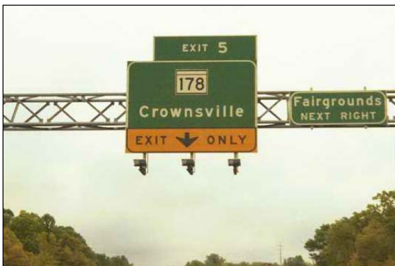
Figure 13 - Box Chord Truss
