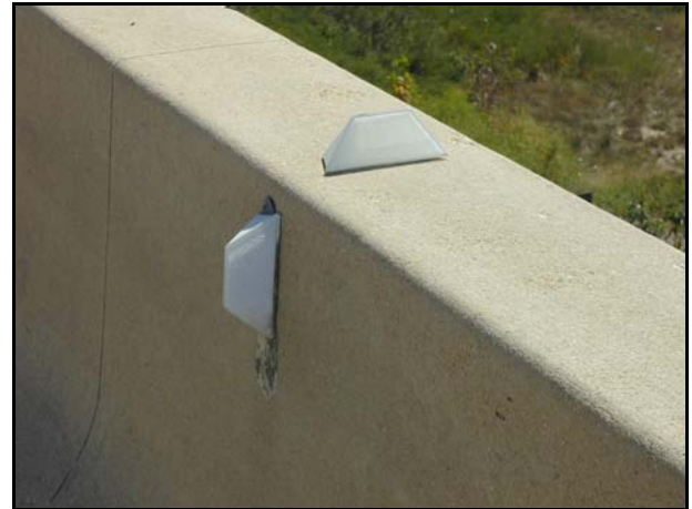
Figure 31 – Top and Side Mounted White Barrier Wall Markers
