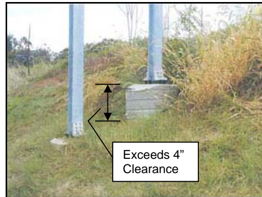
Figure 25 – Improper Supports on Steep Slopes
