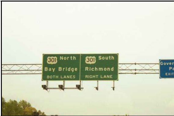
Figure 12 - Tri-Chord Truss
