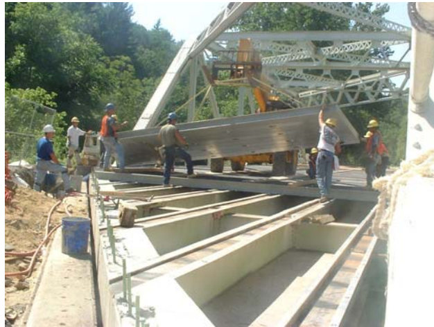
Figure 5.1 – Placement of a FRP Deck Panel
