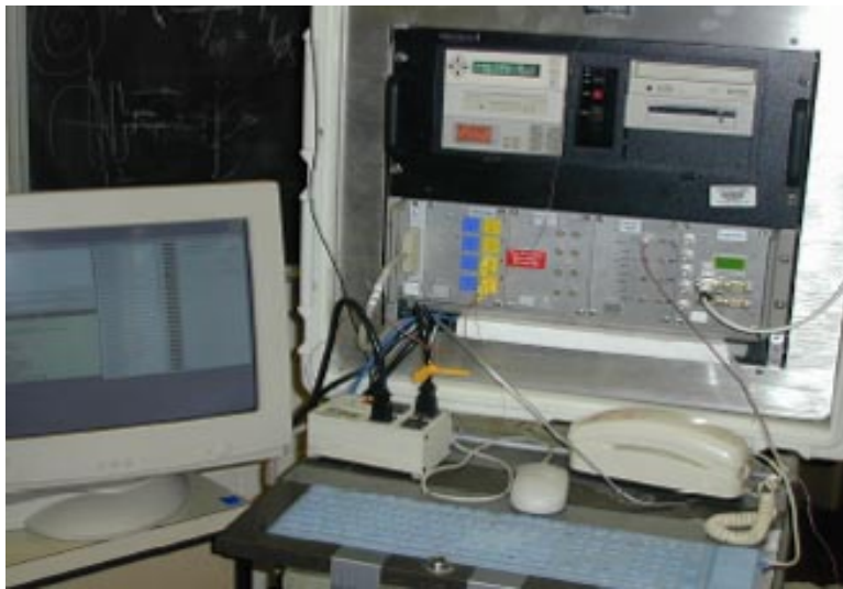
Fielded components of the monitoring system
