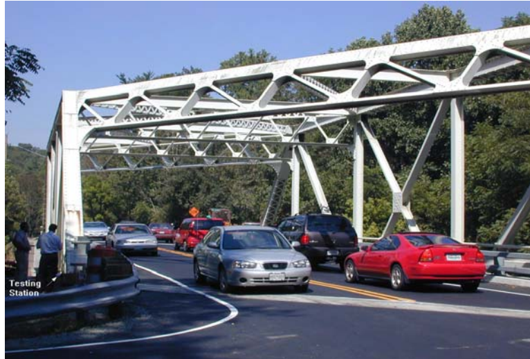
Figure 5.3 - Bridge Testing Calibration of the New FRP Deck under Live Load
